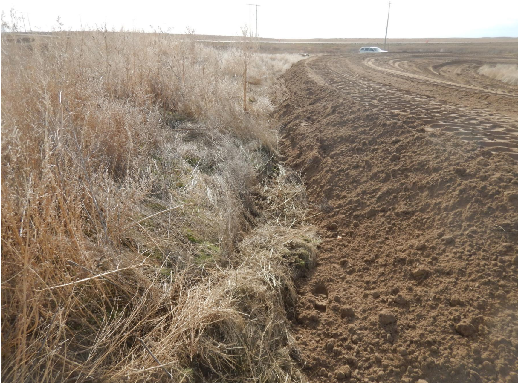
Figure 4: Photo taken from topsoil berm on east end of location, facing south. Photo shows insufficient stormwater BMPs in place.
