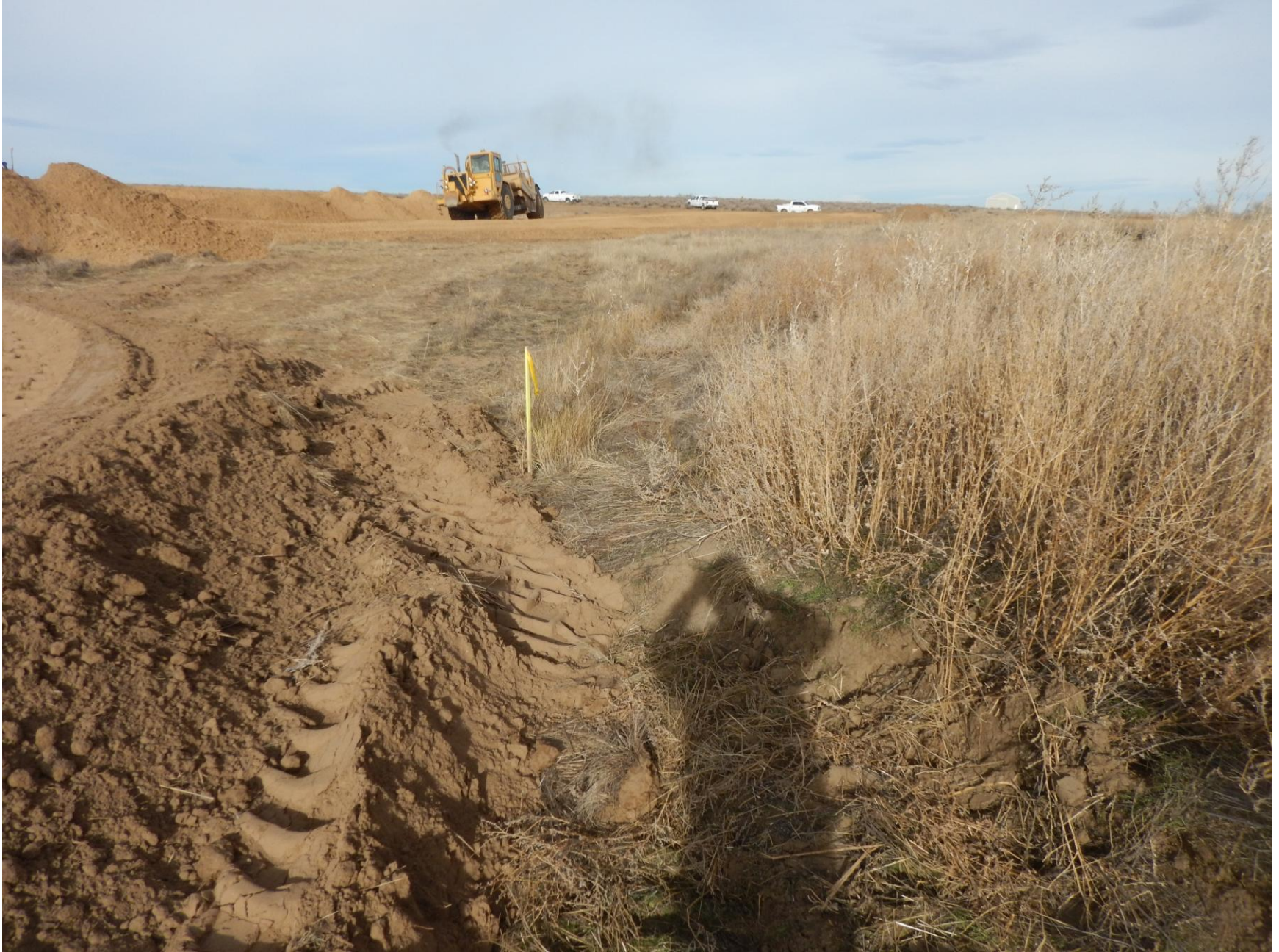
Figure 5: Photo taken from topsoil berm on east end of location, facing northwest. Photo shows insufficient stormwater BMPs in place.
