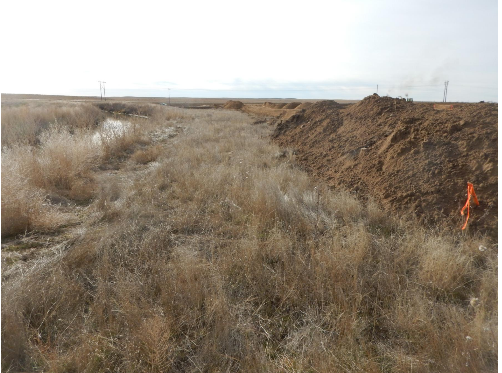
Figure 9: Photo taken from northeast end of location, facing south. Photo shows insufficient stormwater BMPs. Please note irrigation ditch on left of photo.
