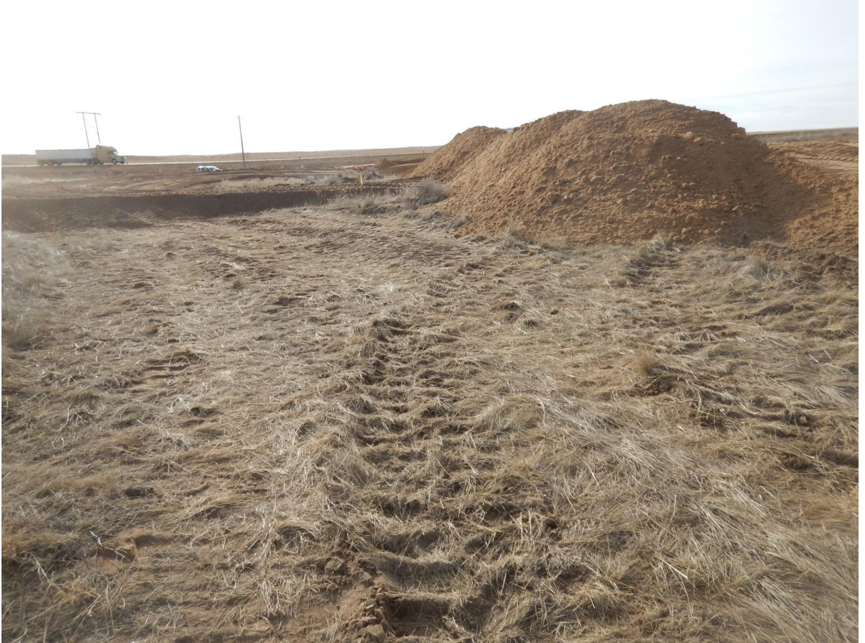
Figure 6: Photo taken from east end of location, facing south. Photo shows insufficient stormwater BMPs in place.
