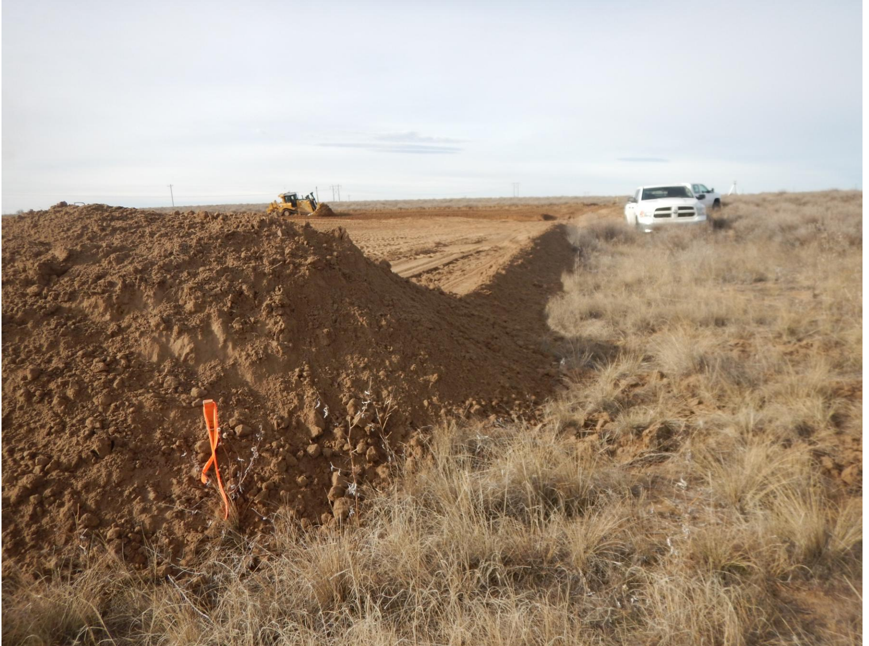
Figure 10: Photo taken from northeast end of location, facing west. Photo shows insufficient stormwater BMPs.
