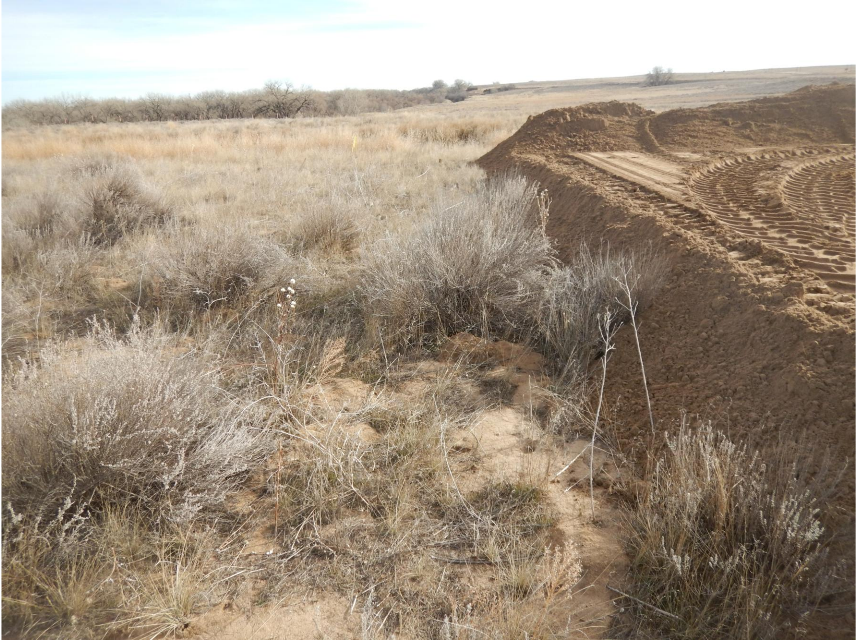
Figure 11: Photo taken from north end of location, facing east. Photo shows insufficient stormwater BMPs.
