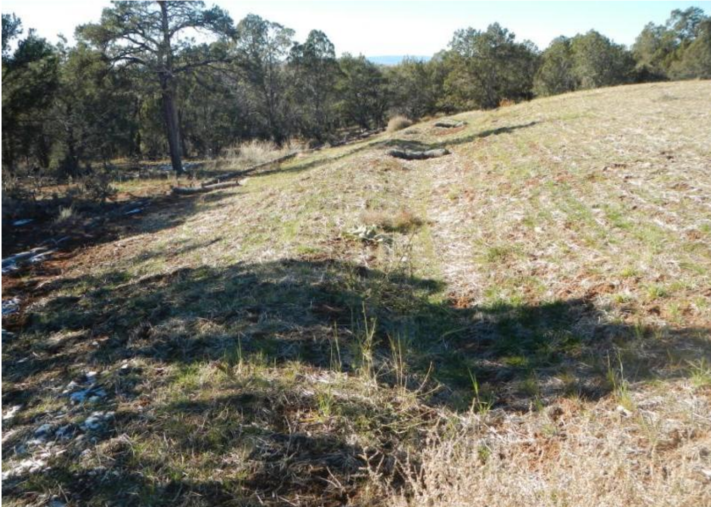
Photo 3. View of the western portion of the project area facing northward. Straw wattles are in place along the stormwater diversion channel and revegetation is progressing.
