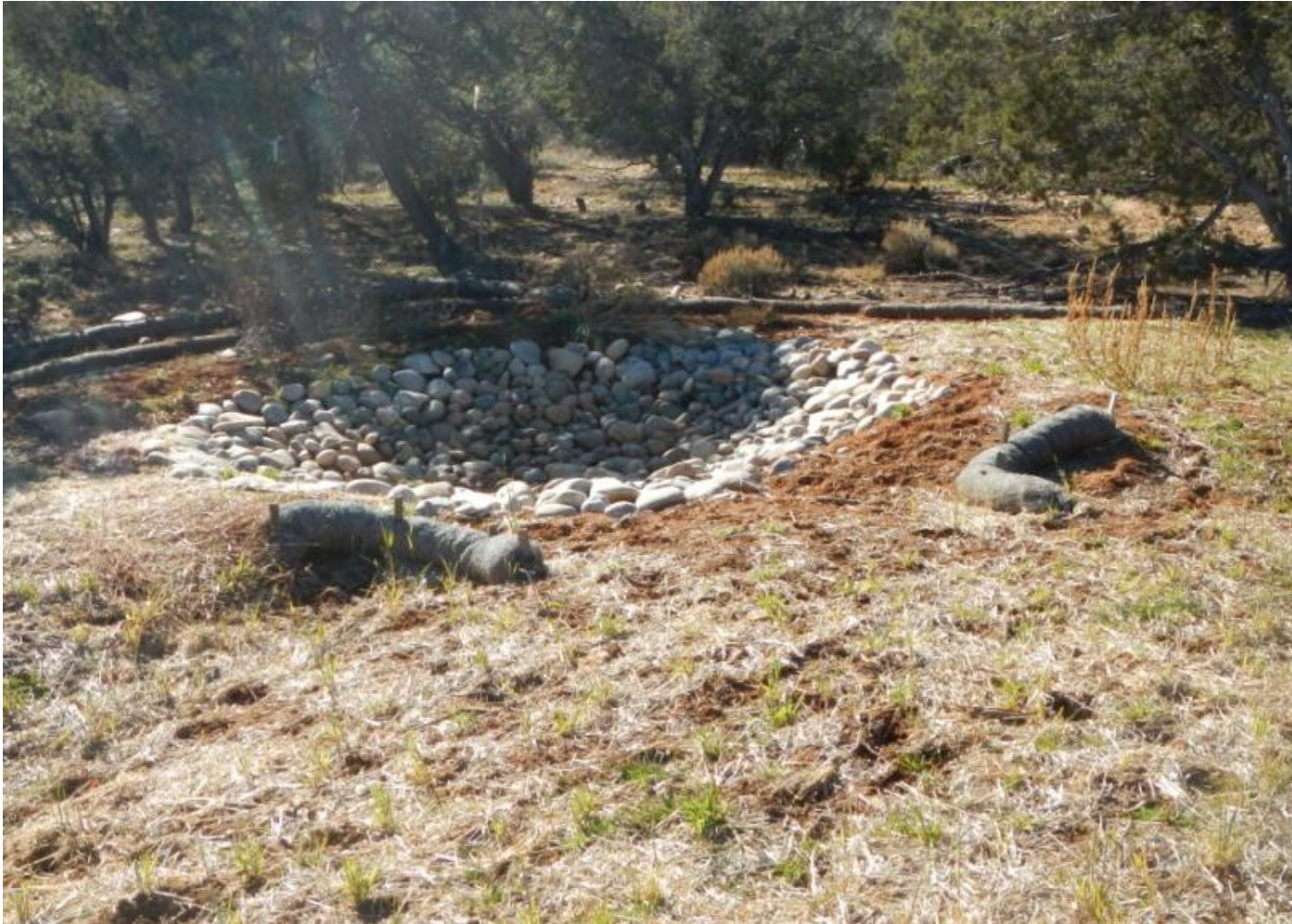
Photo 4. View of cobble lined silt trap and wattles appear to be in good condition within the southwestern corner of the project area.
