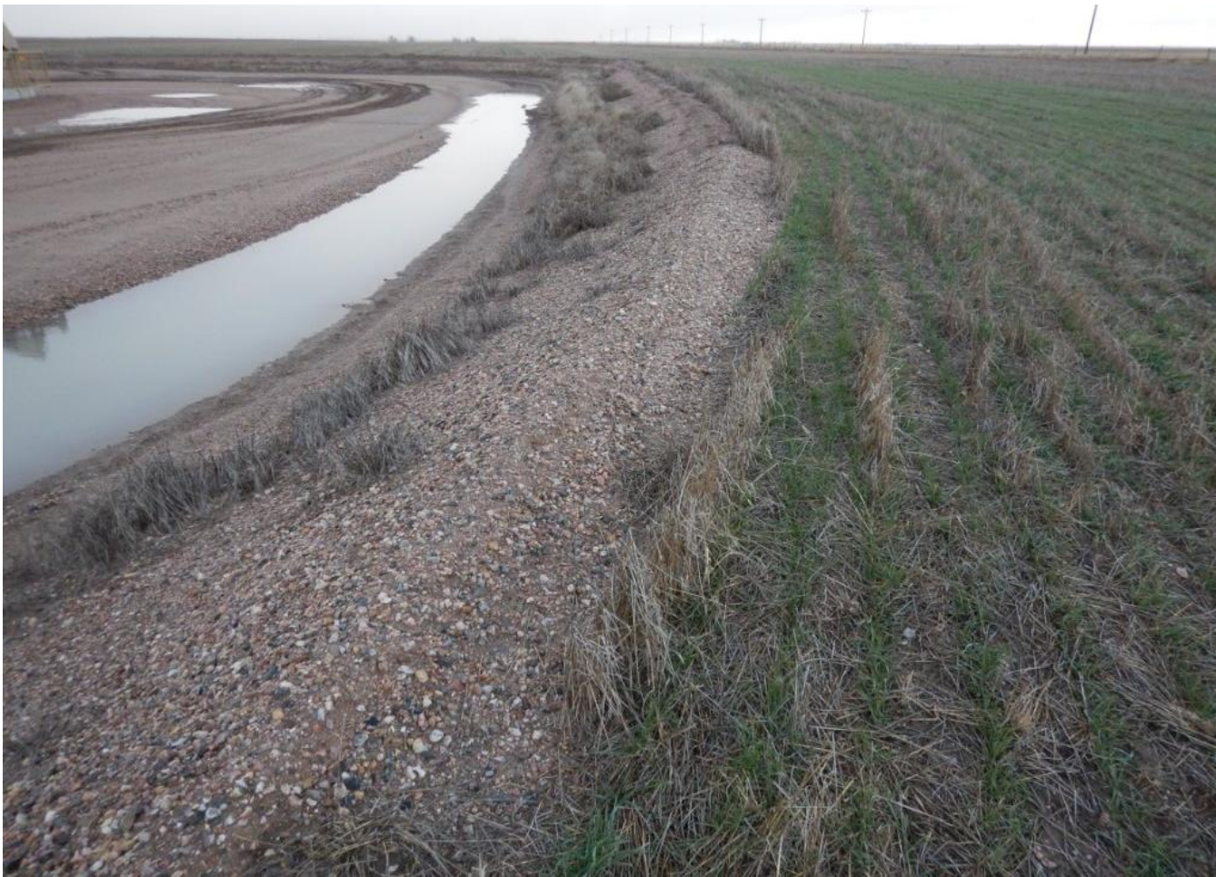
Photo 5. Photo taken from southeast corner, facing North. No noxious weed present and contoured back to agricultural field. Water pooling present along perimeter of well pad.
