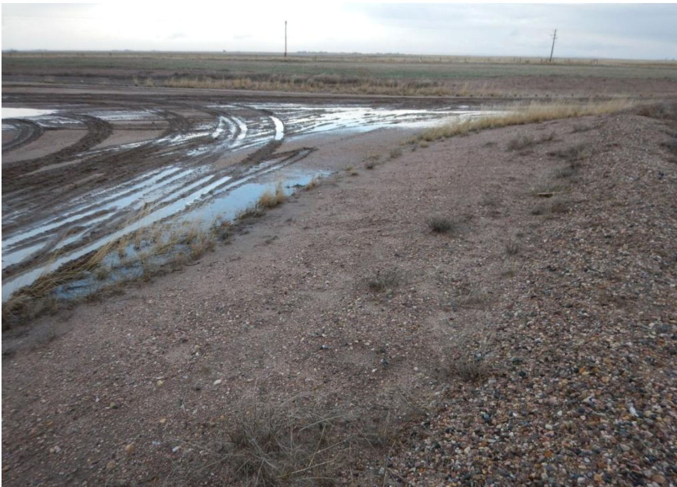
Photo 3. Photo taken from southwest corner, facing East. No noxious weed present and contoured back to agricultural field. Water pooling present along perimeter of well pad.
