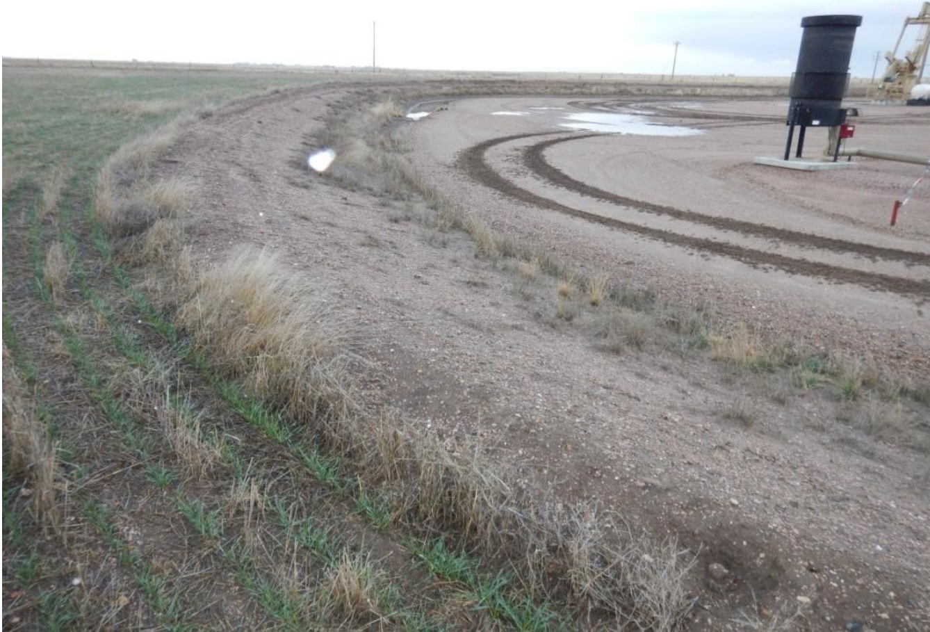
Photo 2. Photo taken from northwest corner, facing East. No noxious weed present and contoured back to agricultural field. Water pooling present along perimeter of well pad.
