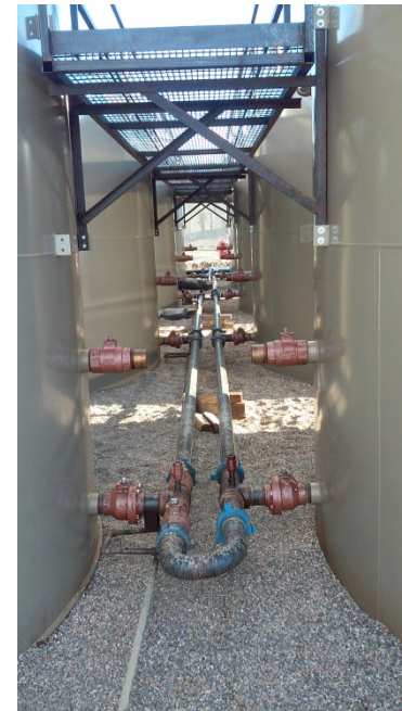
Contaminated material has been removed and new gravel spread.
