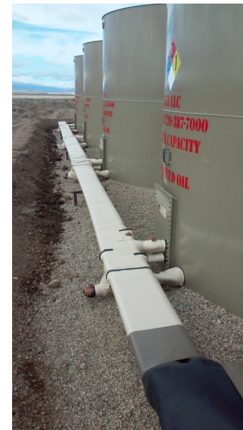
Berm has been raised and liner secured.
