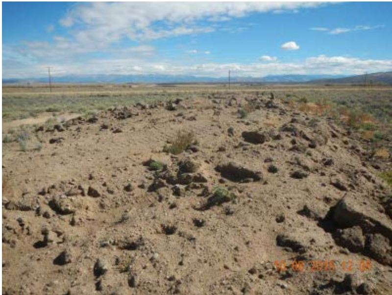
Topsoil pile on south side of location with no visible protection or preservation.
