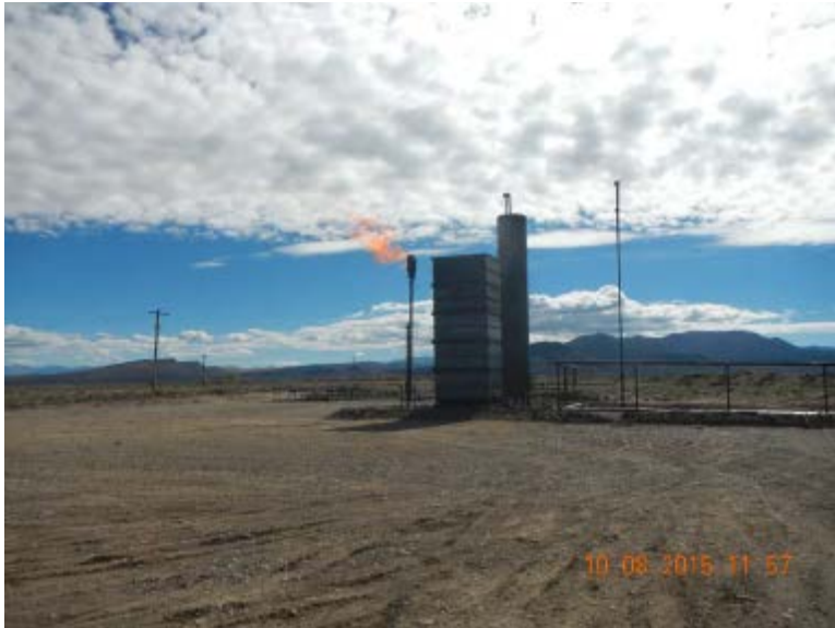
One enclosed flare, 1 unenclosed flare; both lit.
