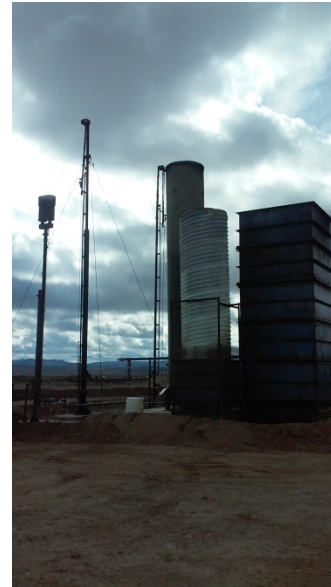
Unenclosed flare is no longer used, all gas is flared in enclosed flare.
