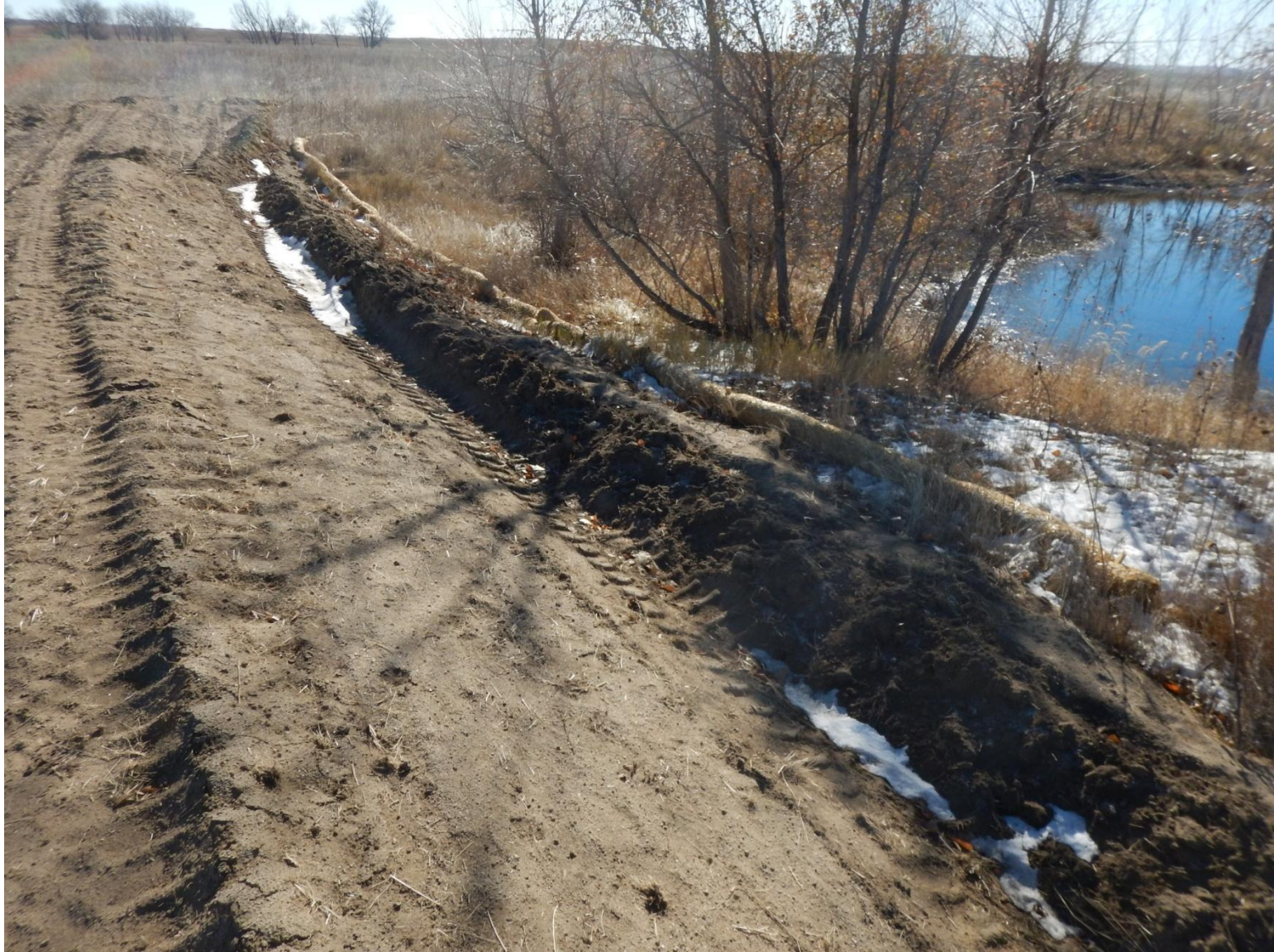
Photo 2: Photo taken from south end of location .Photo showing topsoil berm and tertiary stormwater BMPs.
