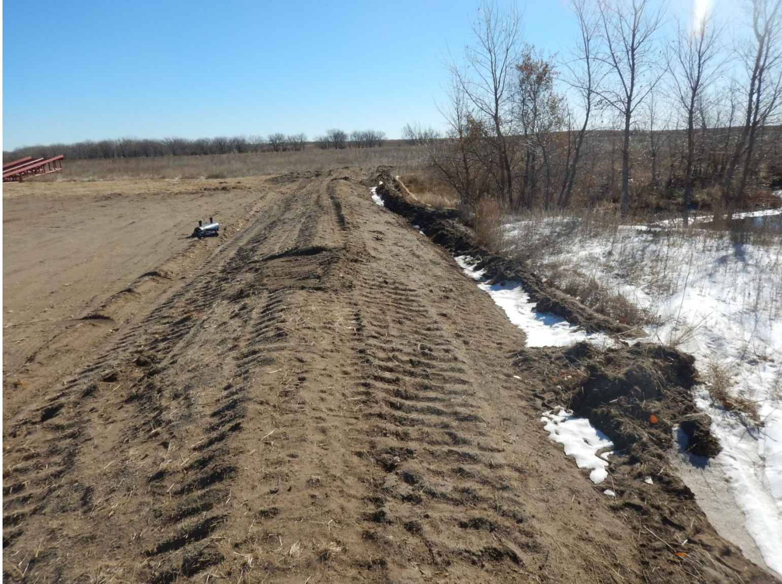
Photo 1: Photo taken from south end of location facing east. Photo showing topsoil berm and stormwater BMPs.
