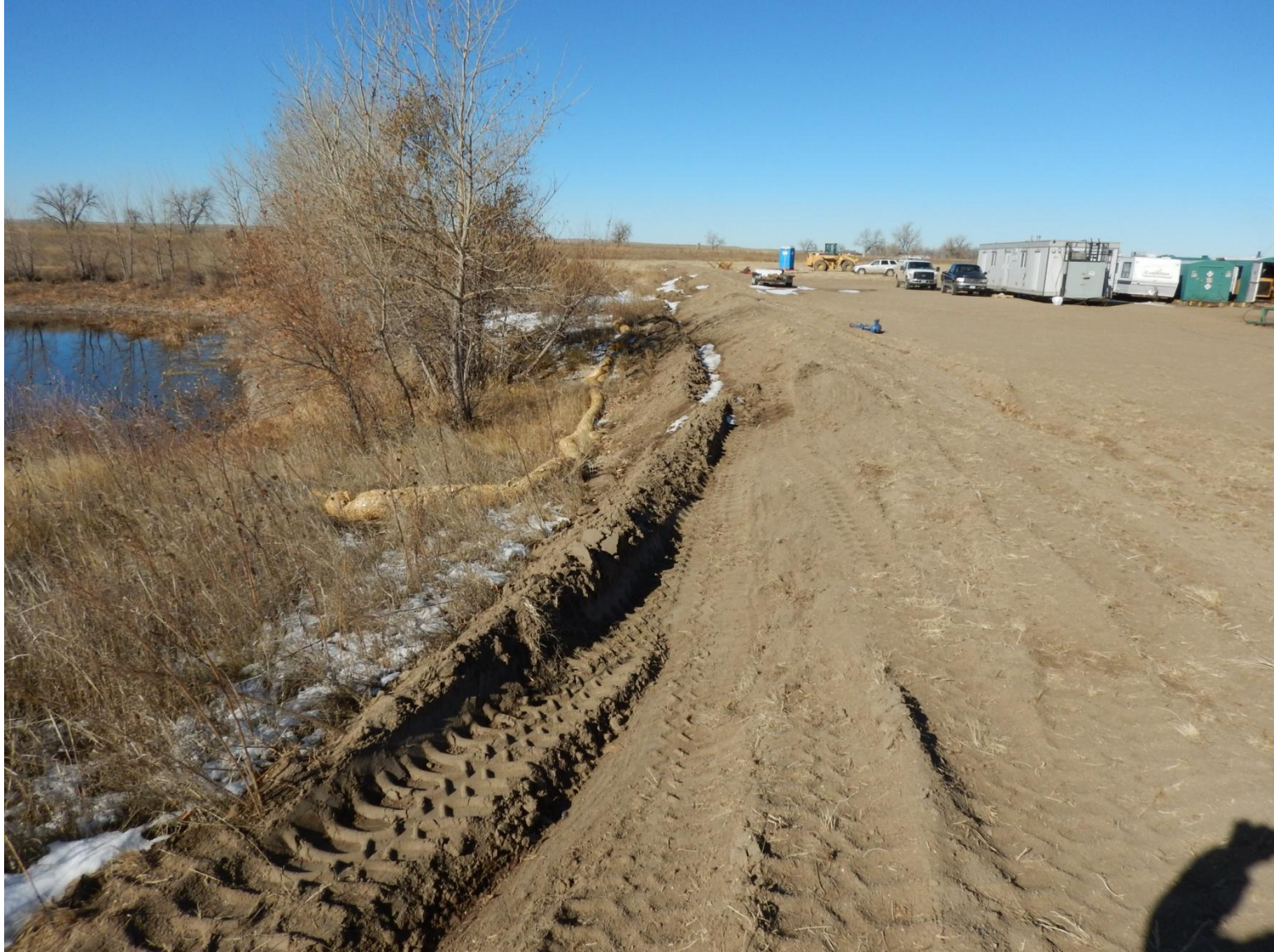
Photo 3: Photo taken from south end of location .Photo showing topsoil berm and tertiary stormwater BMPs. .
