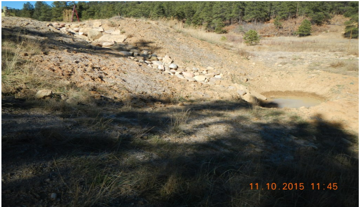
photo 5: East side of the location. Stormwater controls have been installed to prevent erosion.
