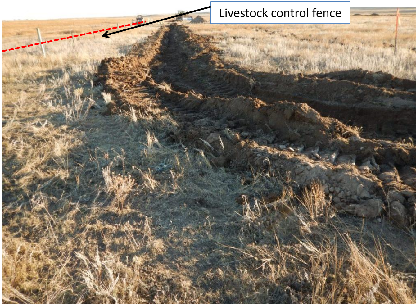
Photo 1. Photo taken from northeast location, facing South. Stormwater control ditch in center of photo. Livestock (cattle) control fence installed around perimeter of disturbance.
