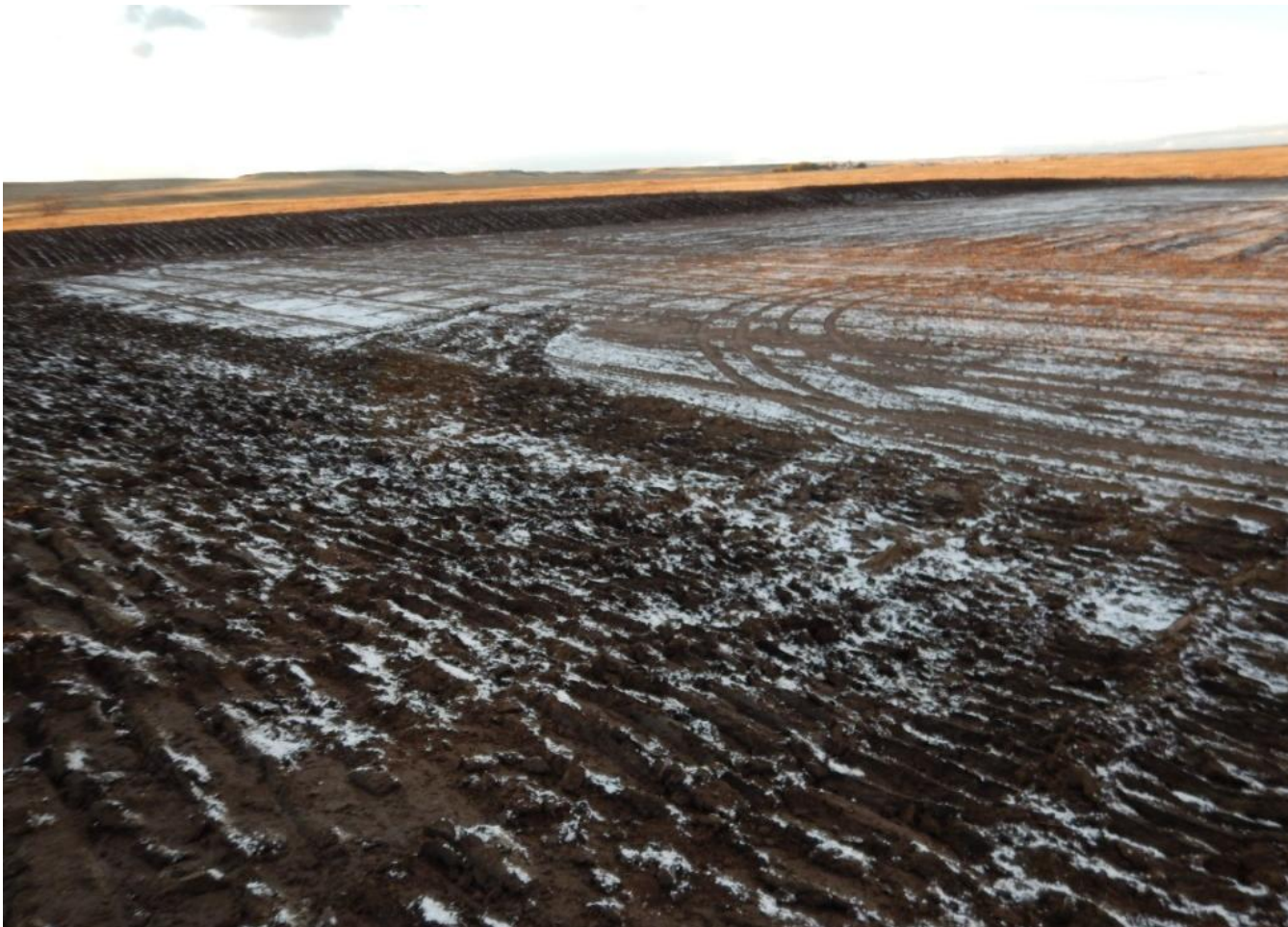
Photo 9. Photo taken from southern location, facing Northwest. Topsoil salvage pile tracked perpendicular to slope.
