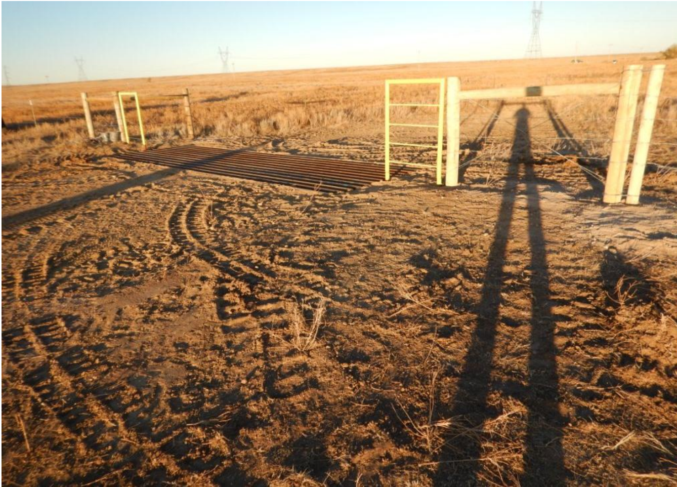
Photo 6. Photo taken from eastern access entrance, facing Northeast. Cattle guard installed in center of photo.
