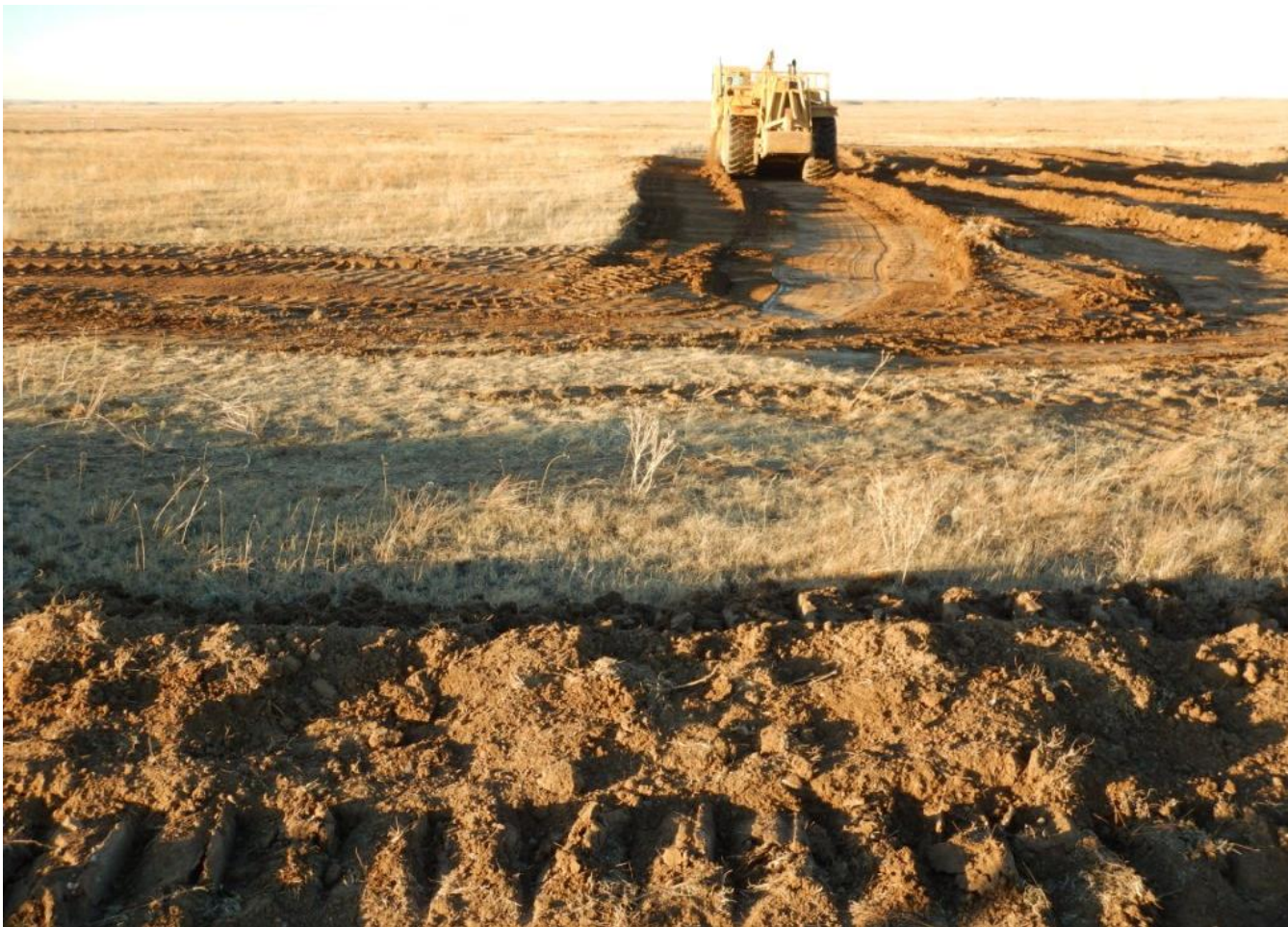
Photo 7. Photo taken from southern location, facing North. Topsoil salvage in process.
