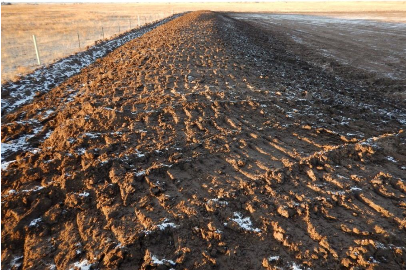
Photo 8. Photo taken from southwest location, facing North. Topsoil salvage pile tracked perpendicular to slope.
