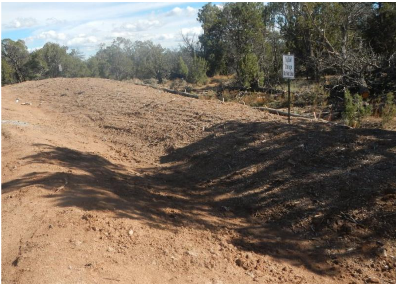
Photo 2. View of southern portion of the project area facing eastward from southwestern corner. Topsoil stockpile is located here. Straw wattles are placed at toe of topsoil stockpile.
