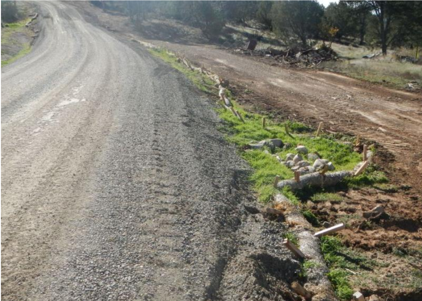
Photo 6. View of access road facing southward. Wattles and cobble armoring are present around culverts and drainage areas.
