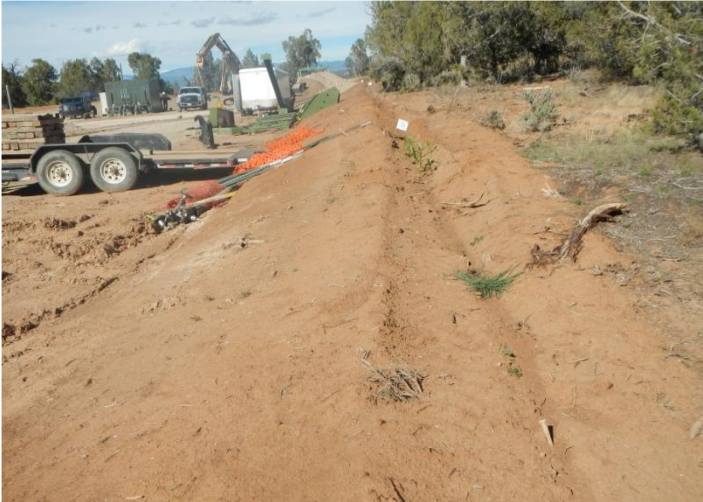
Photo 3. View of eastern portion of the project area from southeastern corner facing northward. Stormwater diversion will need BMPs to prevent downcutting and sediment loss from stormwater flows.
