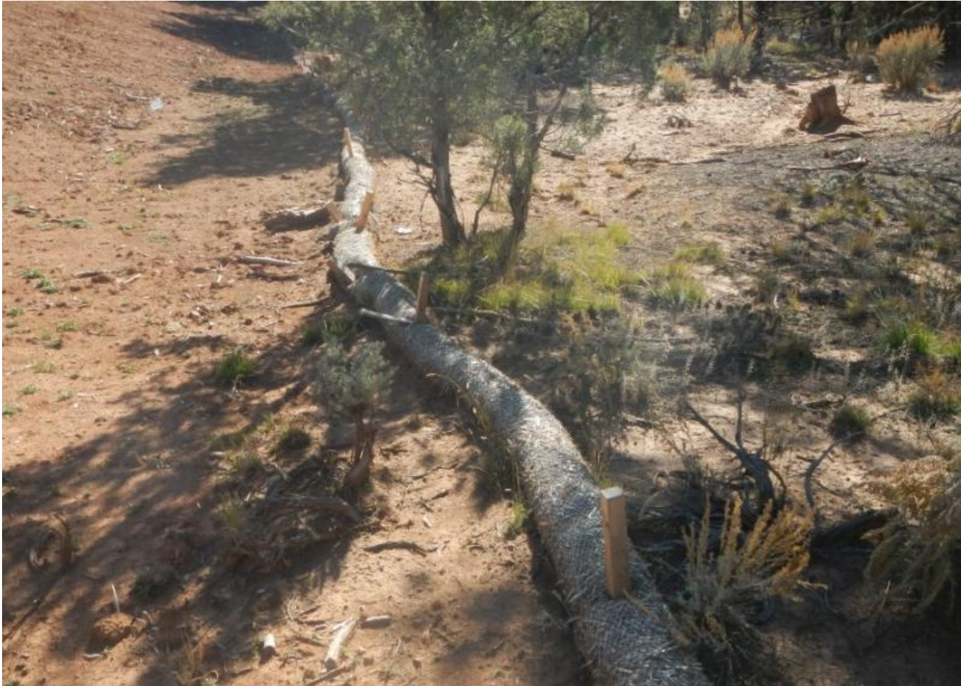
Photo 1. View of straw wattle installed along the western edge of the project area facing southward. Project fill slope located on left side of photo.
