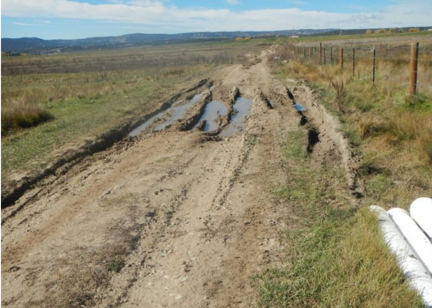
Photo 7. View of ruts (approximately 18 to 20 inches deep) along the access road. It is apparent that vehicles have been driving around to avoid the mud and ruts, as evidenced by tire tracks outside of the driving area.
