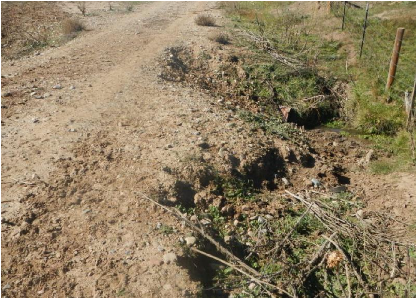
Photo 8. View of erosion occurring around a culvert along the access road.
