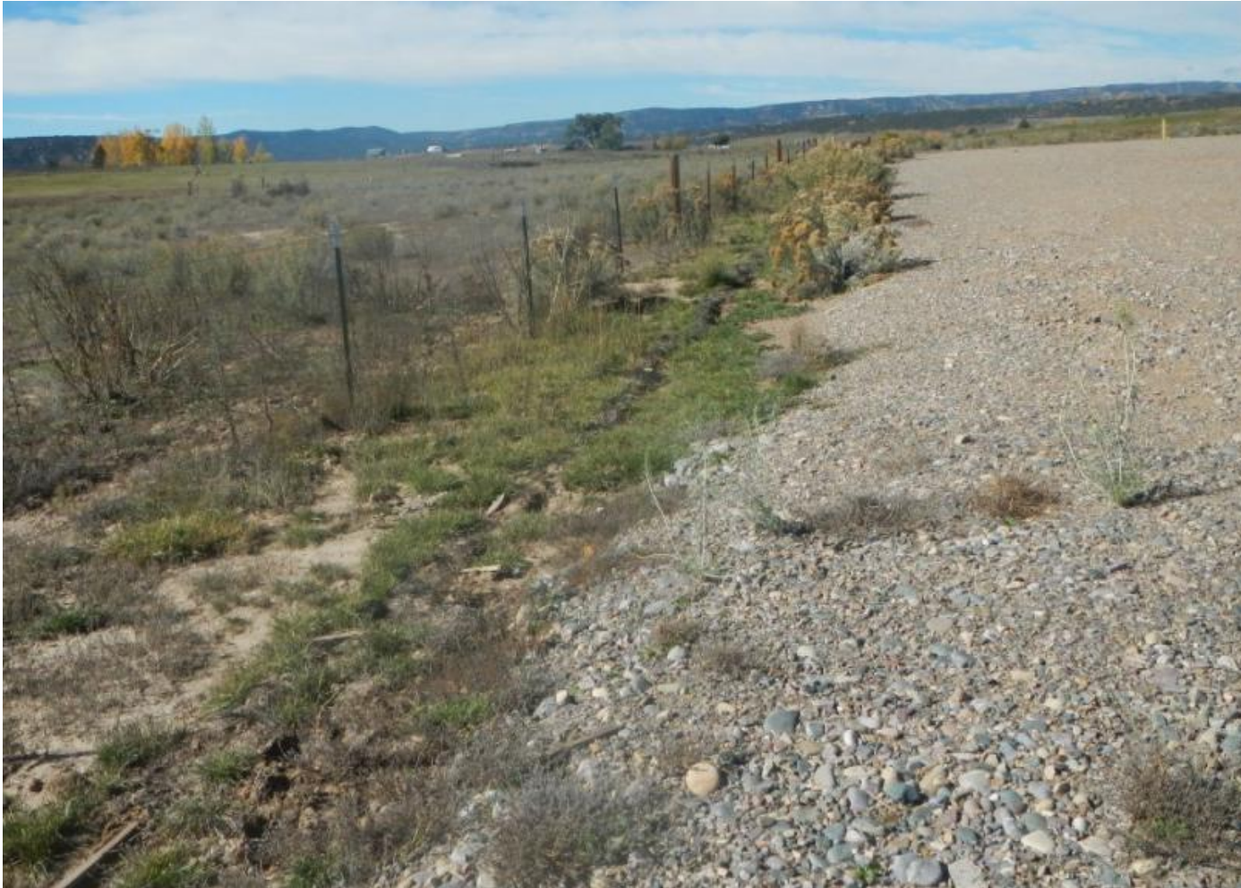
Photo 4. View of southern portion of project area from southeastern corner facing westward. Straw wattle is in disrepair, but vegetation and cobble on the slopes appear to be effectively reducing erosion.
