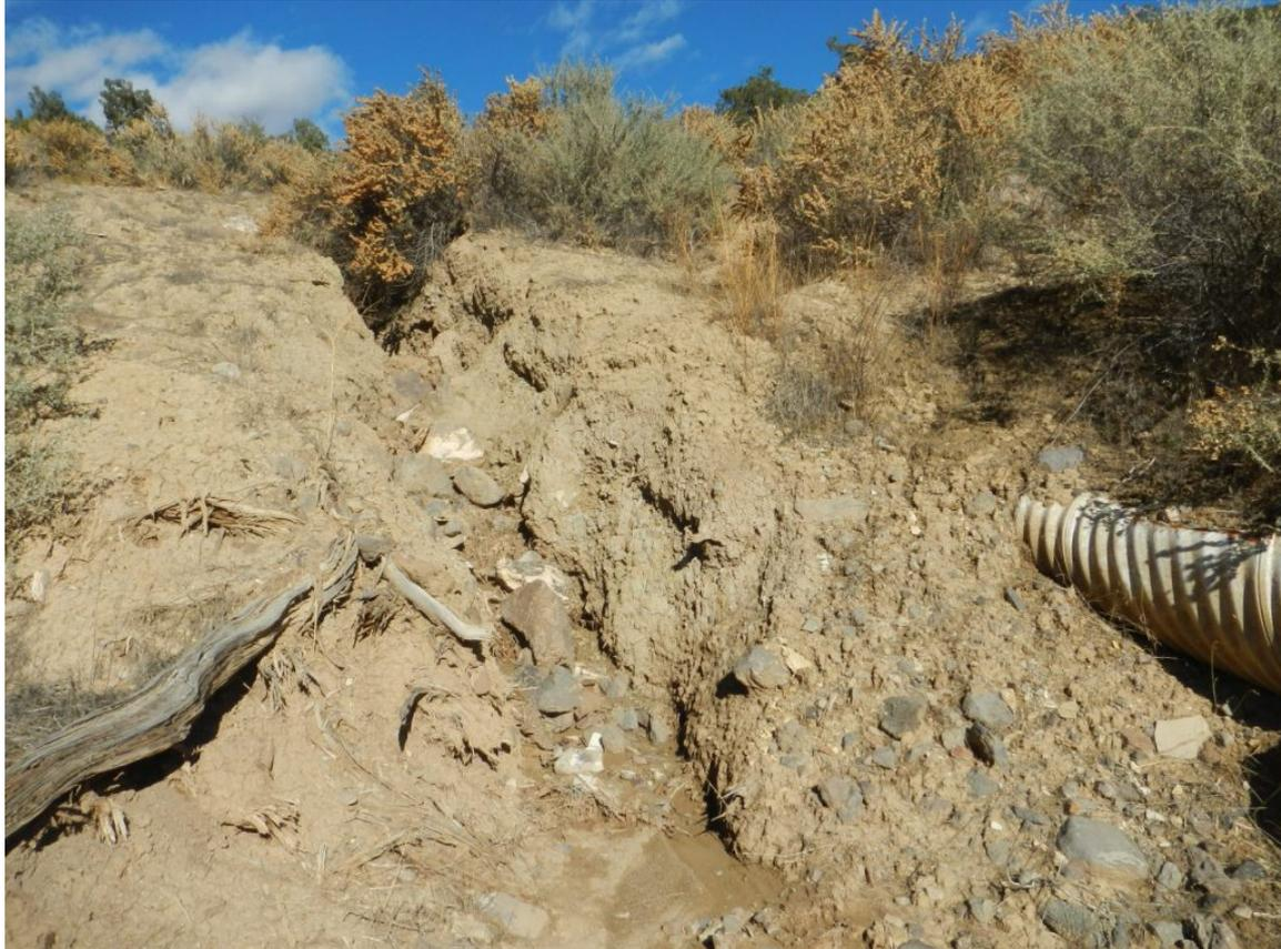
Photo#4: Termination of Gully , exposed undercut culvert at right.
