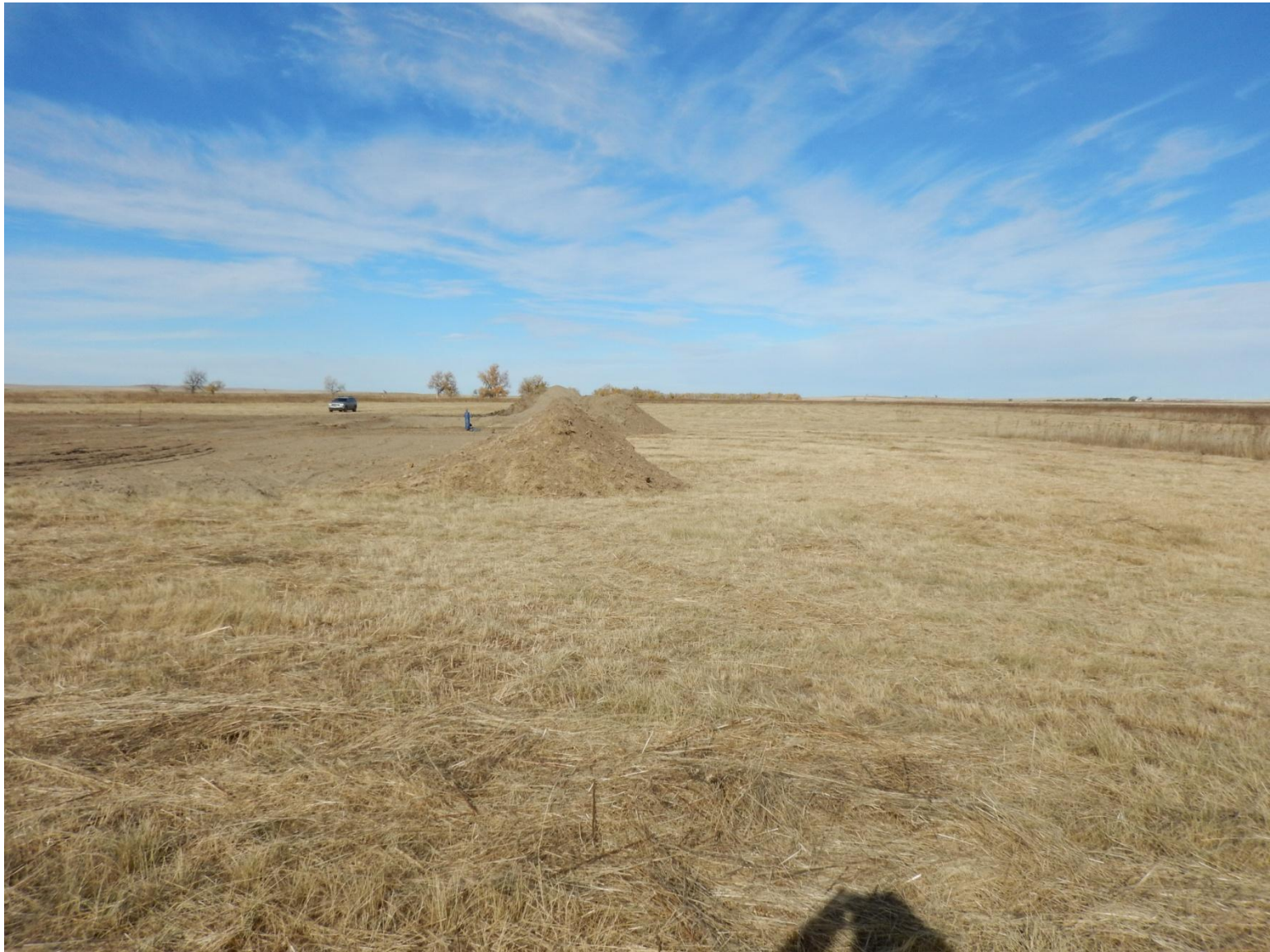
Photo 8: Photo taken from Northeast side of location facing West. Note insufficient storm water BMPs in place along the North side of location.
