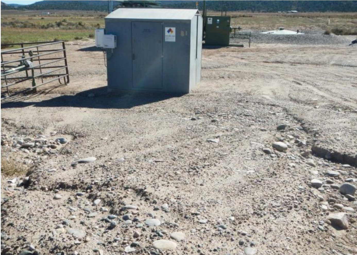
Photo 3. Another view of stormwater erosion in the eastern portion of the project area. Erosional channels are flowing beneath and through project facilities.
