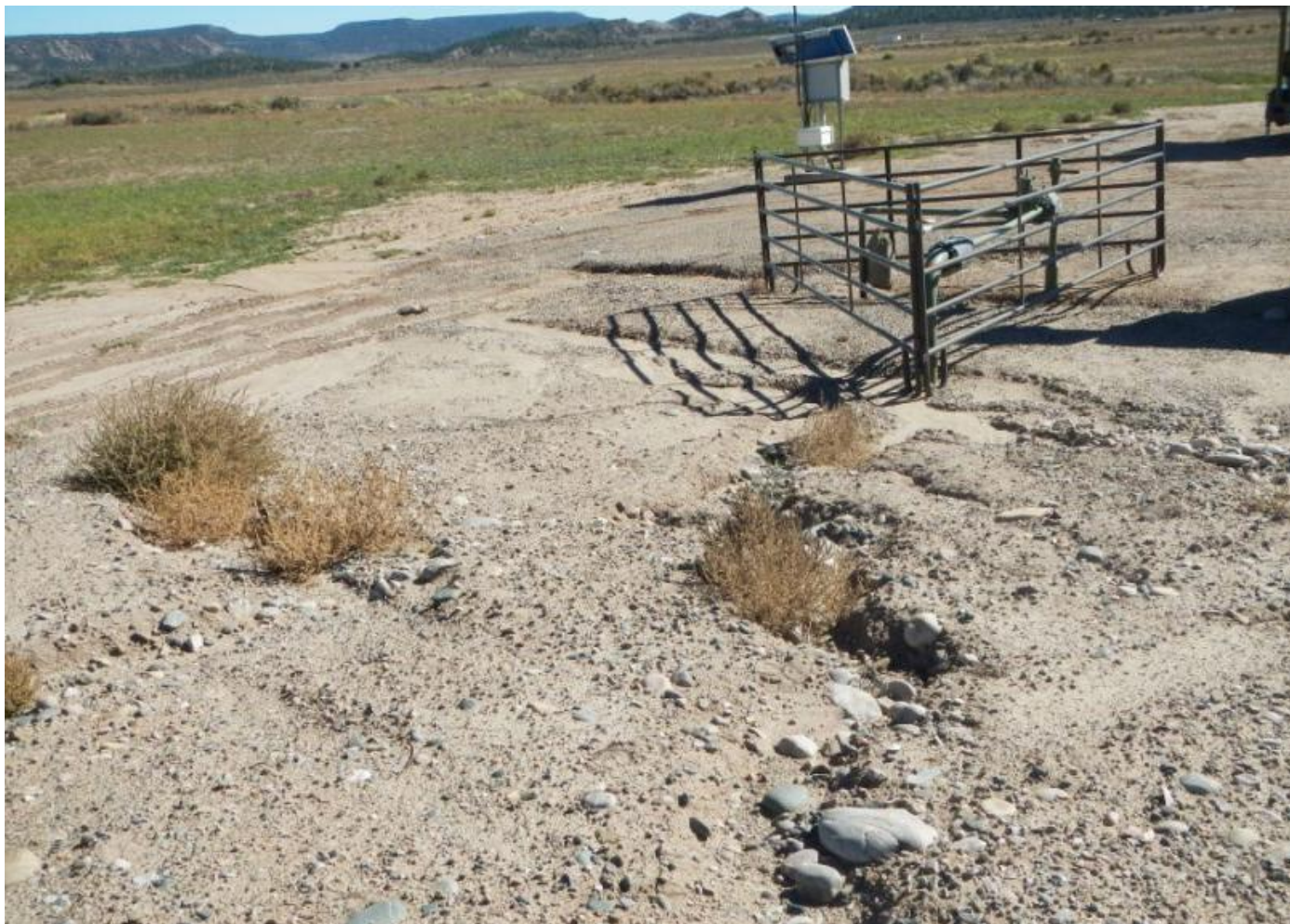
Photo 2. View of stormwater erosion in the eastern portion of the project area. Erosional channels are formed (approximately 12 inches deep and 24 inches wide) and appear to be carrying sediment outside of the project area (in background).
