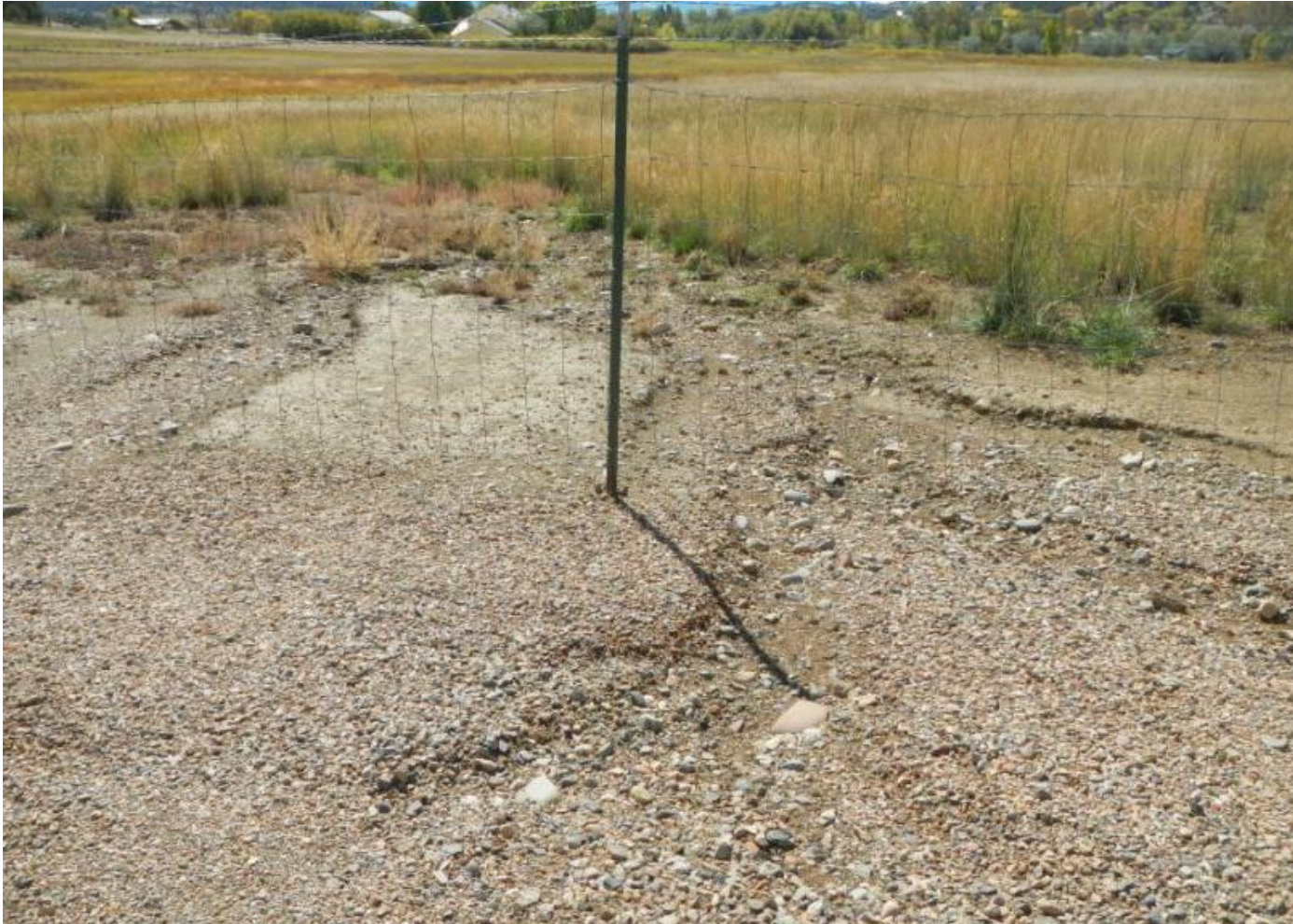
Photo 3. View of southern portion of project area where it appears concentrated stormwater flows are carrying sediment outside of the project area.
