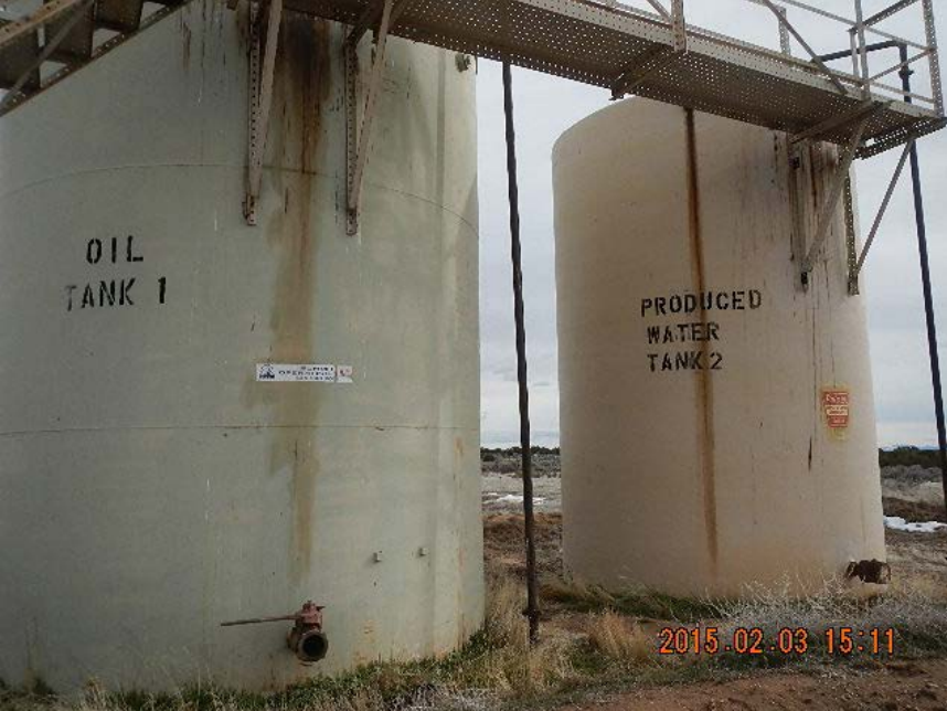
Tank labels missing – initial inspection
