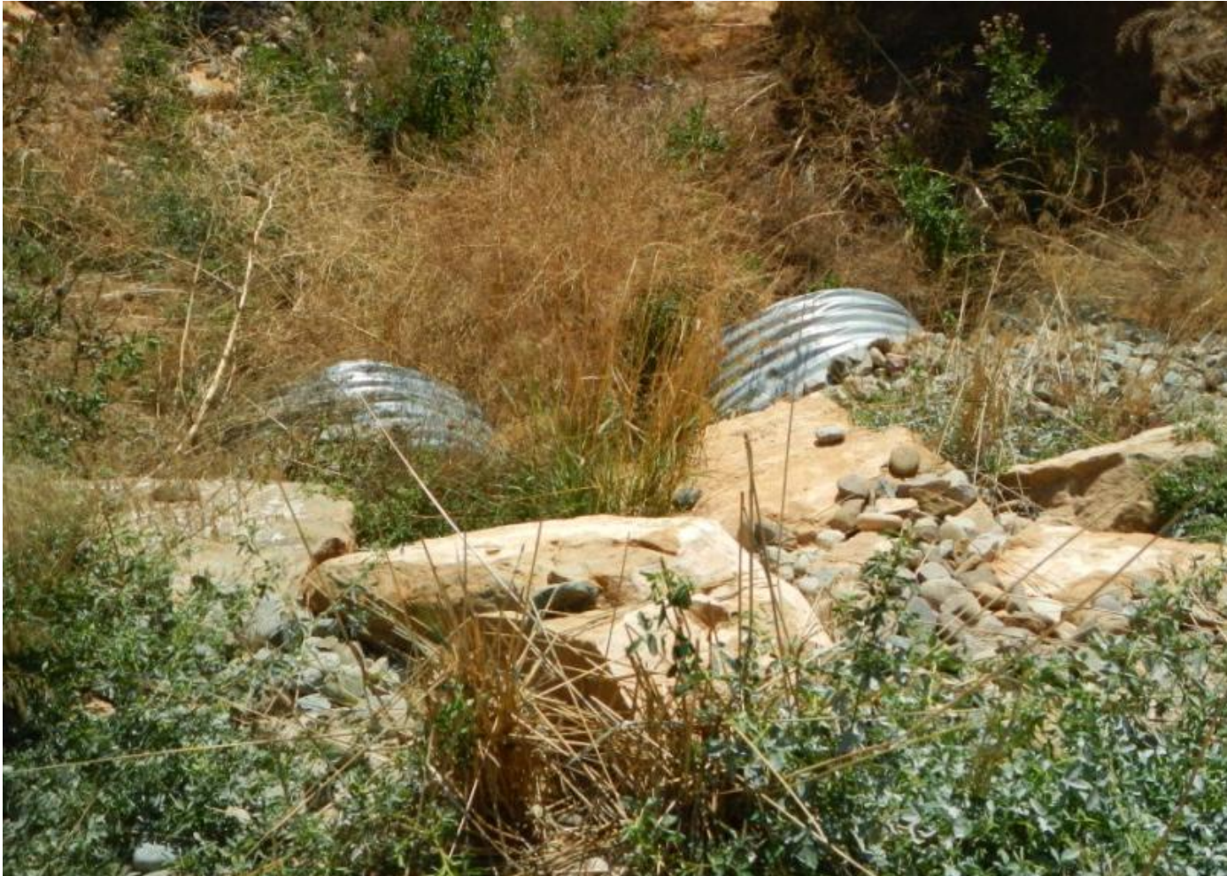
Photo 7. View of rock armor around culverts that appears to be successfully stabilizing potential erosion in this area.
