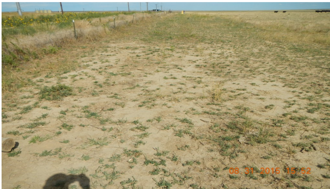
photo 8: Areas along the pipeline in the pasture south of the location have not been properly reclaimed.
