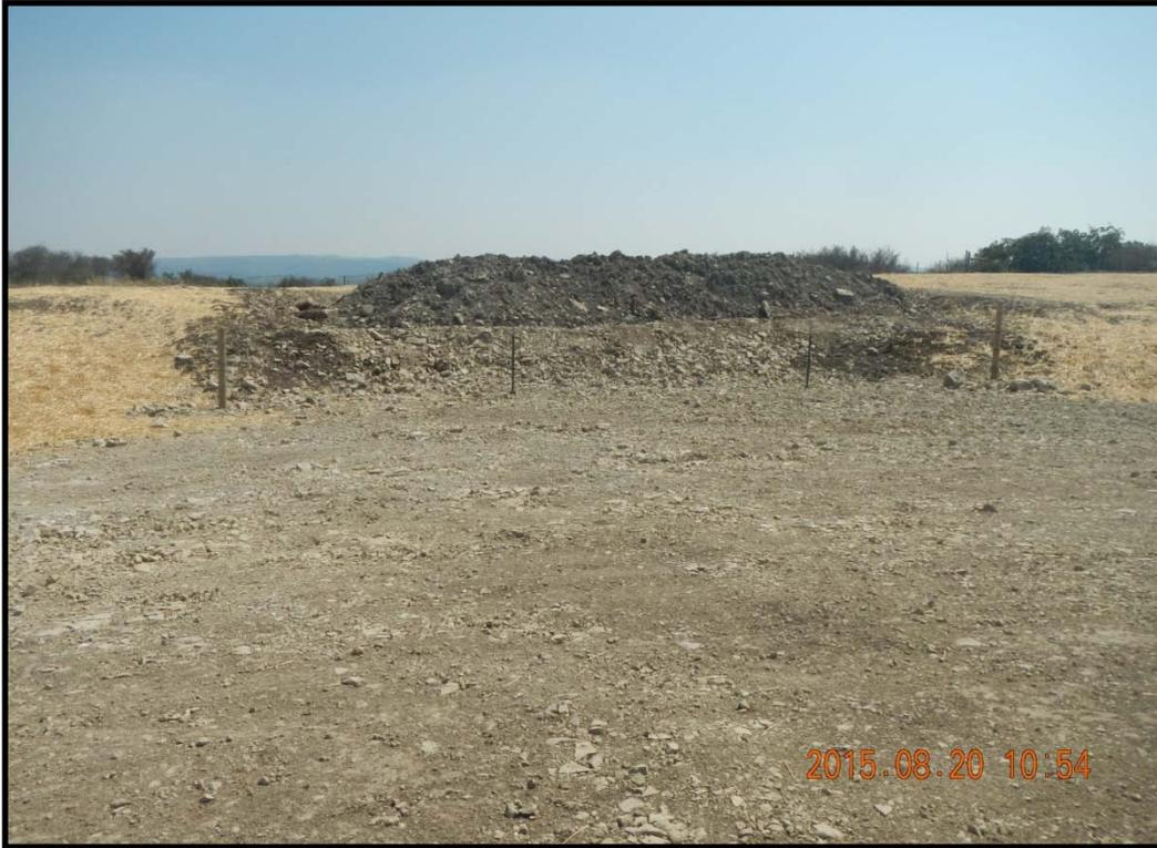
Bermed stockpile of impacted material. According to Linn representative, Derek Johnson, this material comes from the pit recently closed and is being treated to reduce HC concentrations.
