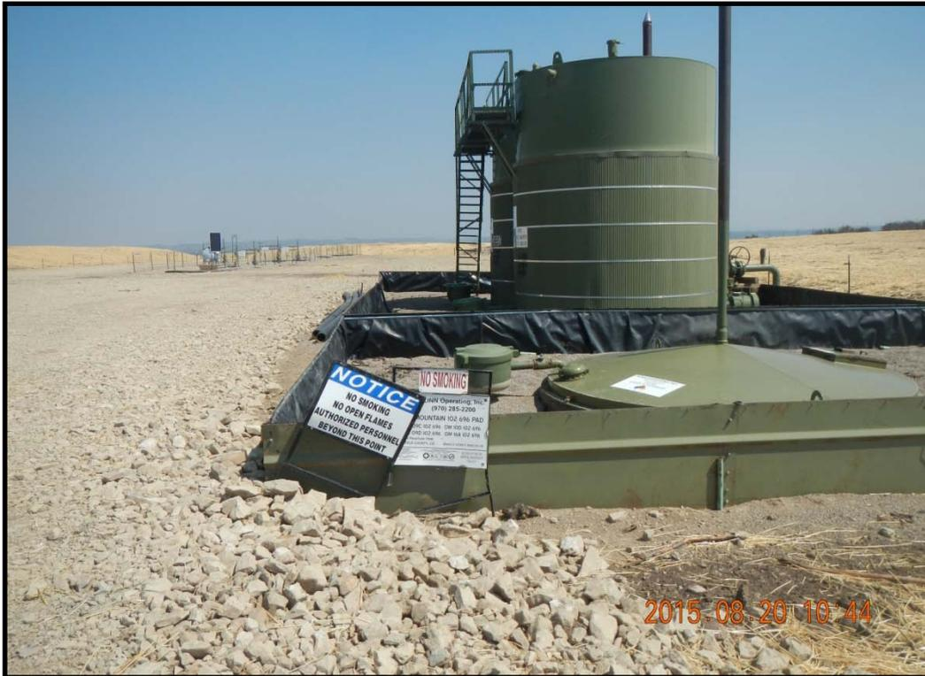
Signs need to be located at the entrance of the pad. Tanks with lined secondary containment.
