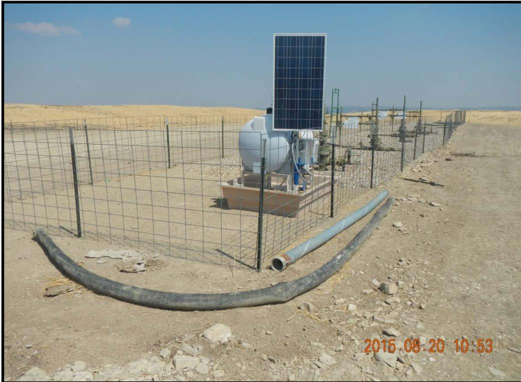
Wellheads area protected with fence. Tubing and pipeline must be removed from Site if not to be used (Housekeeping).
