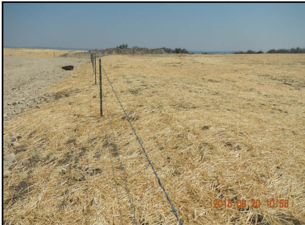
South area of the pad (looking east) reclaimed. Pit ID #415484 has been backfilled, leveled and reseeded.
