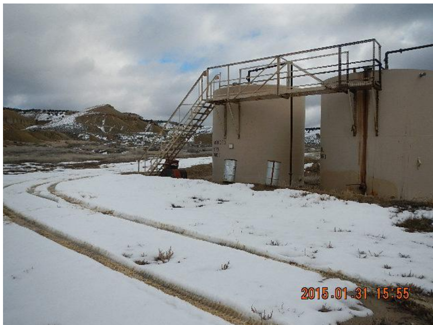
Tanks not labeled and drums – initial inspection
