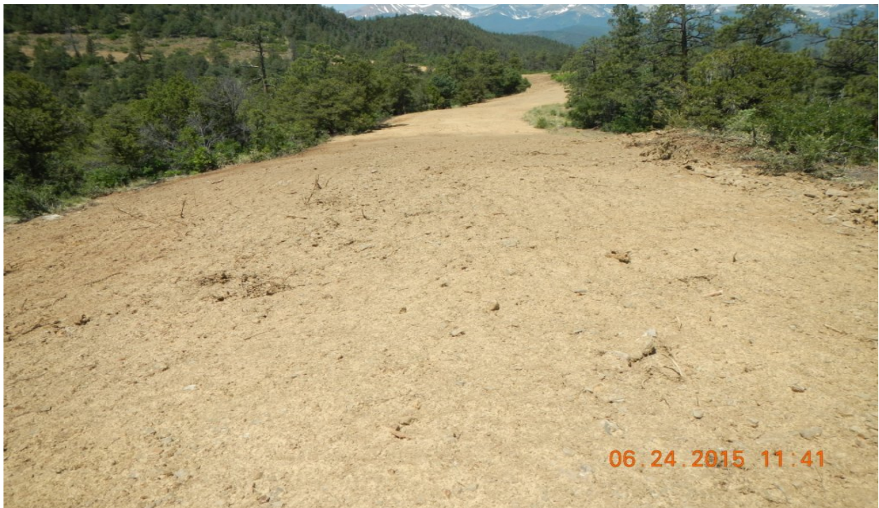
photo 2: Access road facing west towards the location has recently been recontoured and reclaimed.
