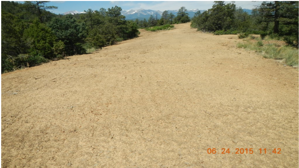
photo 3: Access road facing west towards the location has recently been recontoured and reclaimed.
