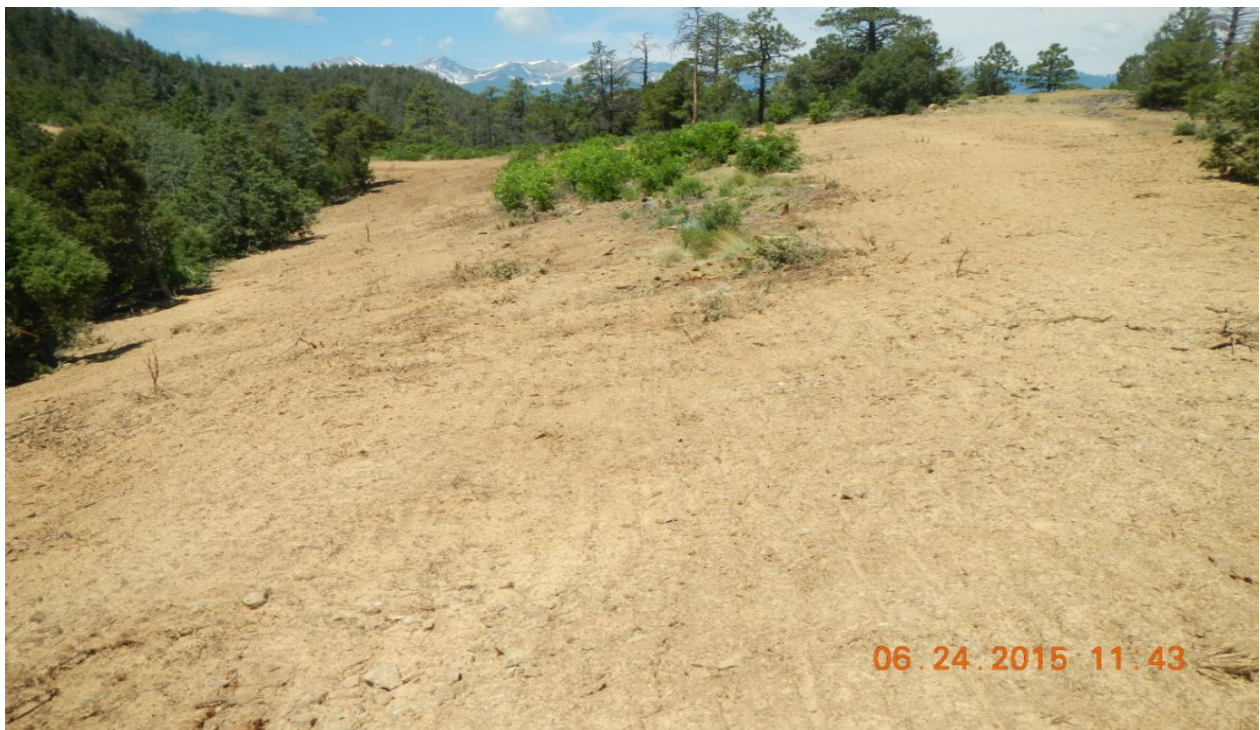
photo 4: Areas of disturbance along the access road have been hydro seeded and mulched.
