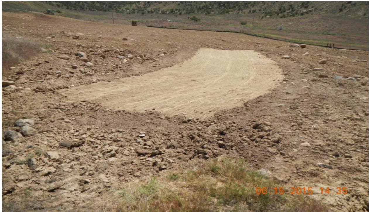
photo 11: A jute blanket was installed at the north side of the location.
