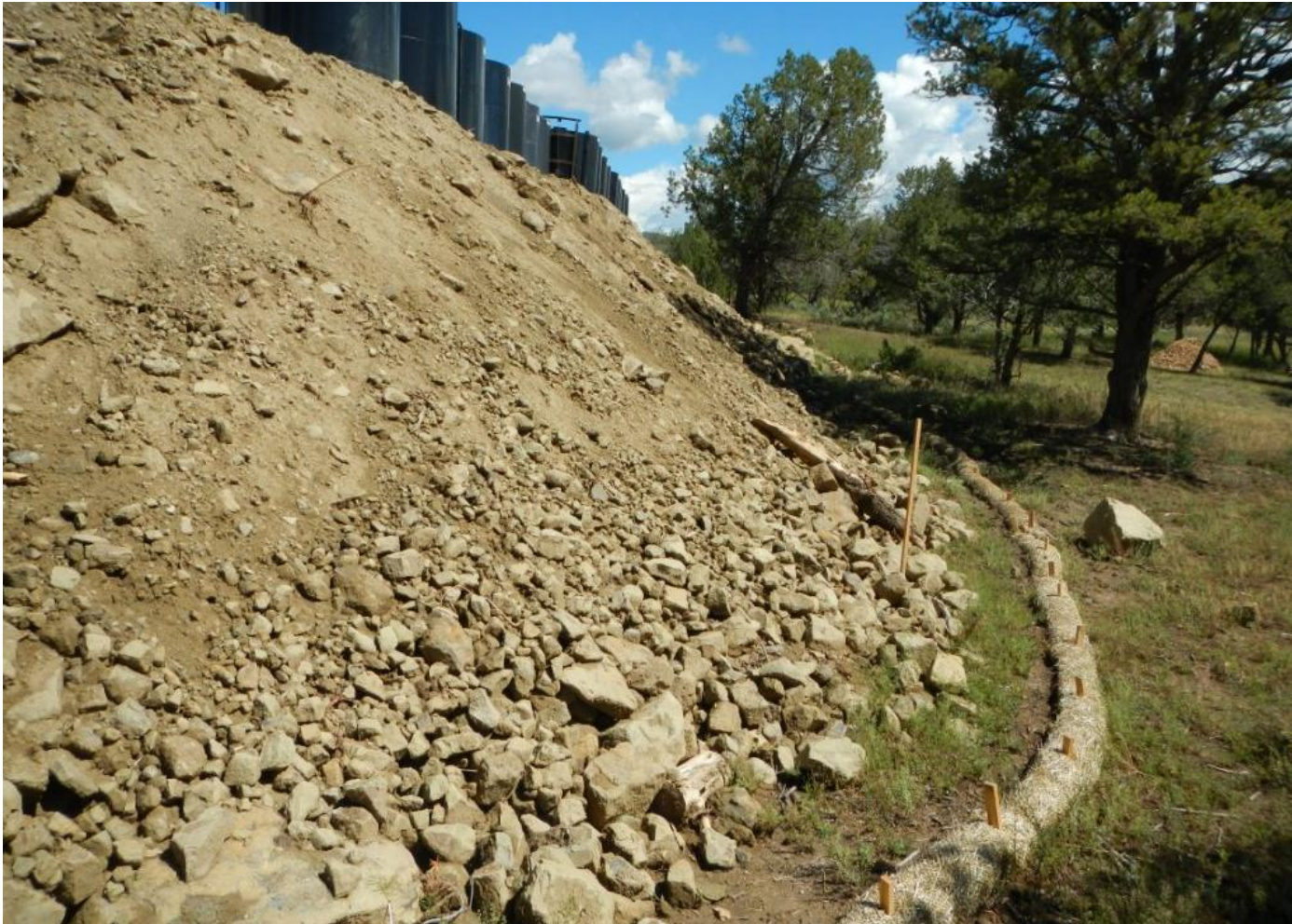
Photo 5. View of eastern edge of project area from southeastern corner facing northward. Perimeter straw wattles appear to be effectively filtering stormwater flows at this time.
