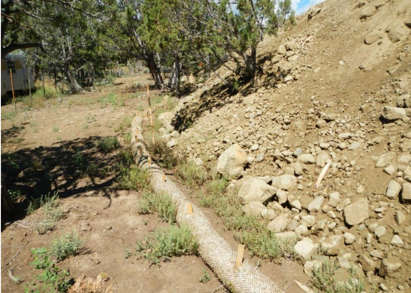
Photo 6. View of southern edge of project area from southeastern corner facing westward. Perimeter straw wattles appear to be effectively filtering stormwater flows at this time.
