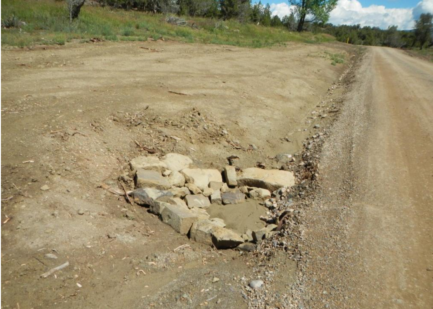
Photo 8. View of culvert inlet along access road. Sediment is accumulating in the inlet basin and will soon need maintenance.
