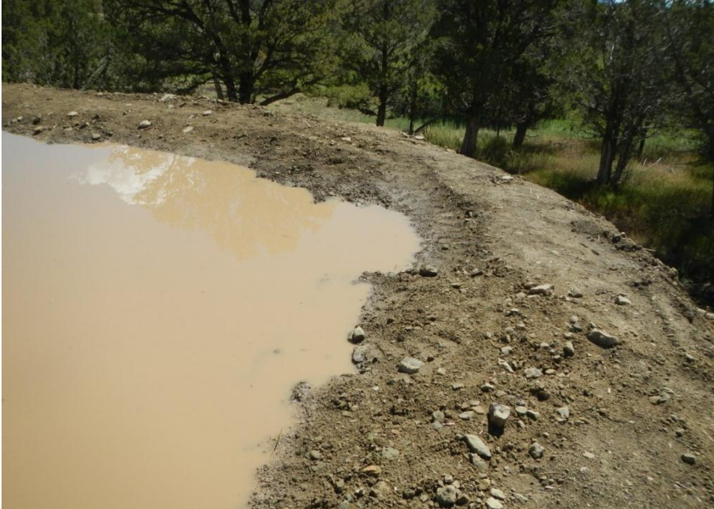
Photo 2. View of stormwater containment in southeastern corner of well pad. This needs to be monitored carefully and deepened and/or reinforced if stormwater continues to accumulate here.
