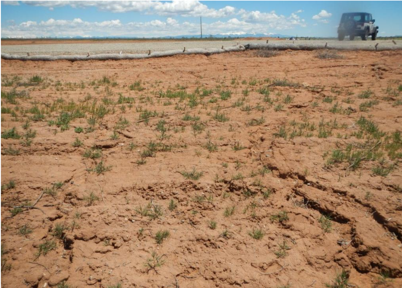
Photo 1. View of rill erosion in western portion of project area, downslope of straw wattles. Vegetation in foreground is largely Russian thistle ( Salsola tragus ).
