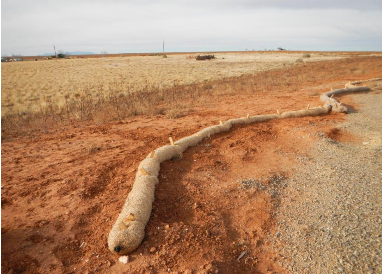
Photo 3. View of straw wattles in western portion of project area.
