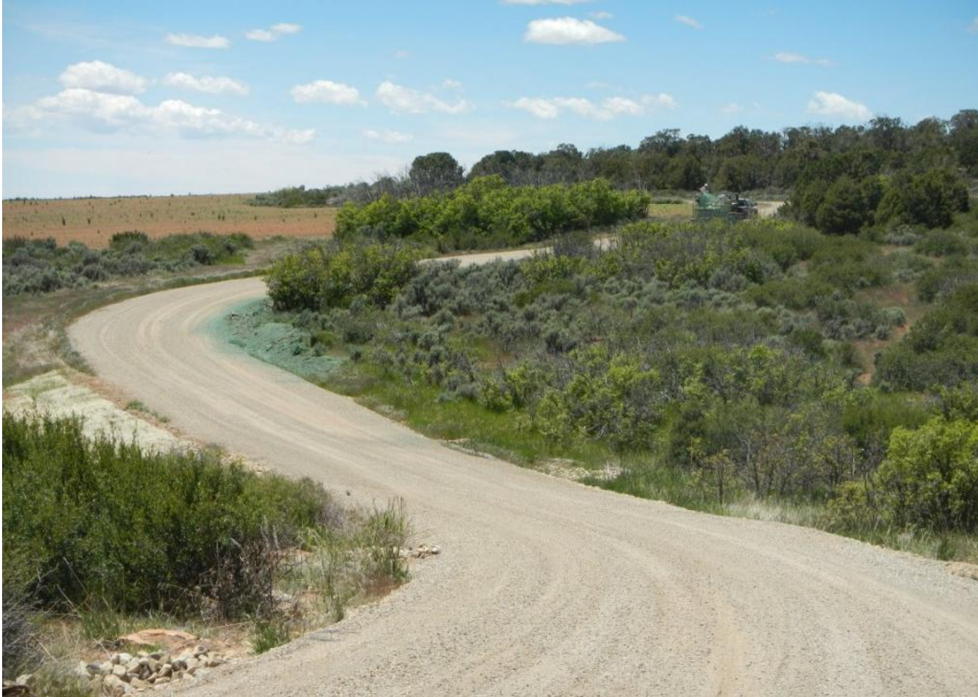
Photo 5. View of hydromulch being applied to the northern edge of the access road.
