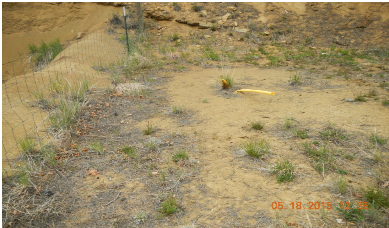
photo 6: The northwest Guyline anchor is not properly marked.
