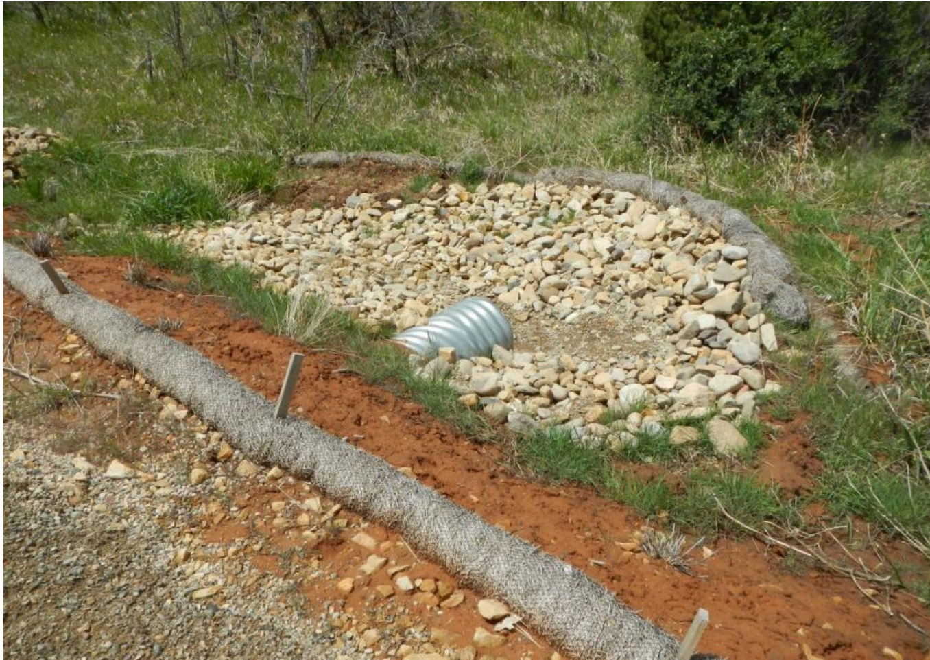
Photo 2. View of functioning BMPS at culvert along access road.
