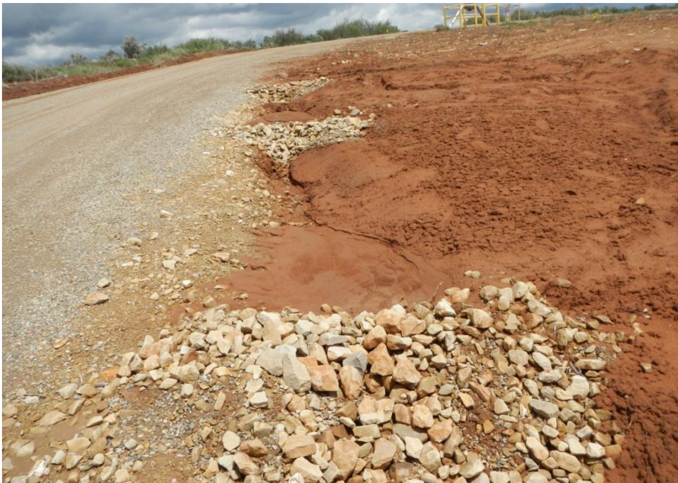
Photo 1. View of stormwater BMPs along access road that will soon require maintenance.
