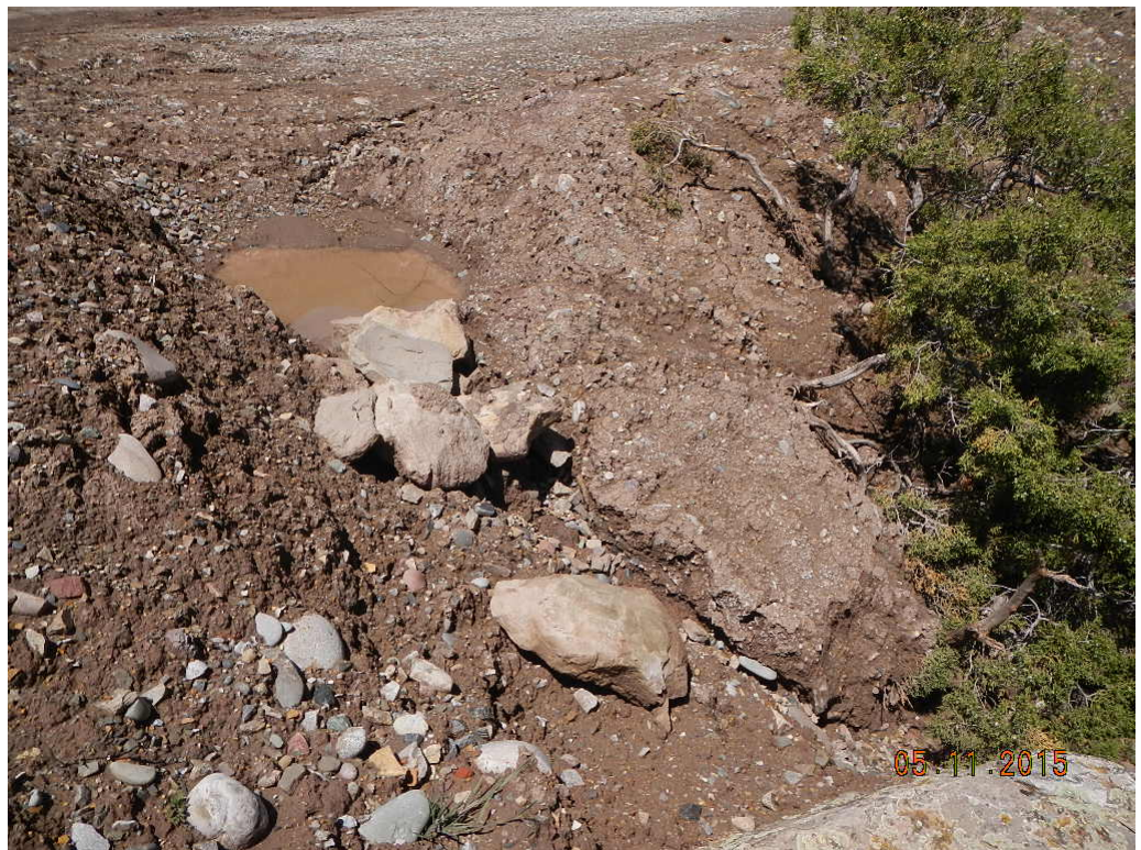
Erosion under rip rap outlet of retention pond.
