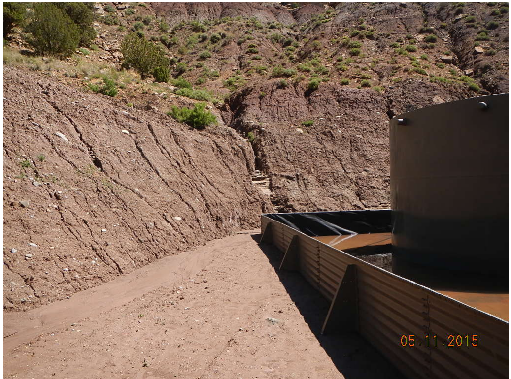
Sediment run on in NE corner of location and erosion channel.
