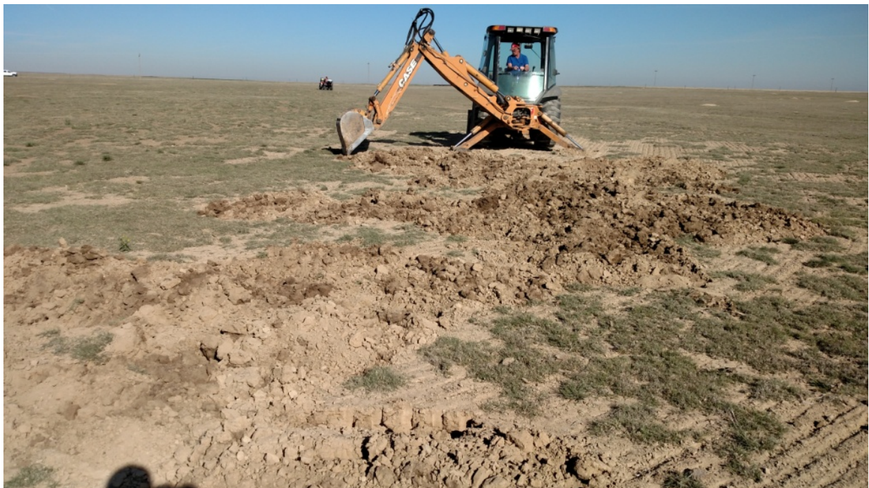
photo 6: Compacted soils being excavated with a backhoe to break up the compacted soils.
