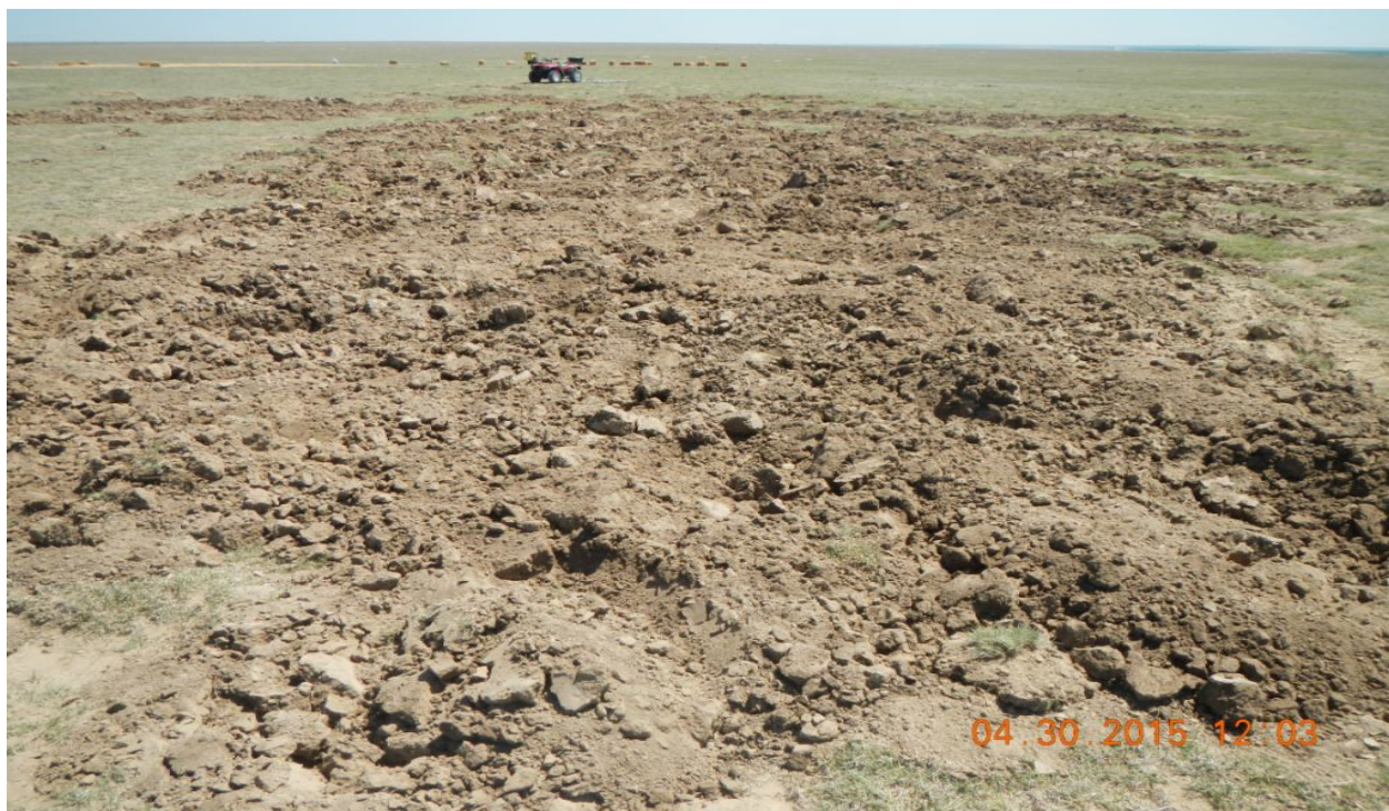
photo 7: Facing east towards areas which were decompacted with the backhoe.
