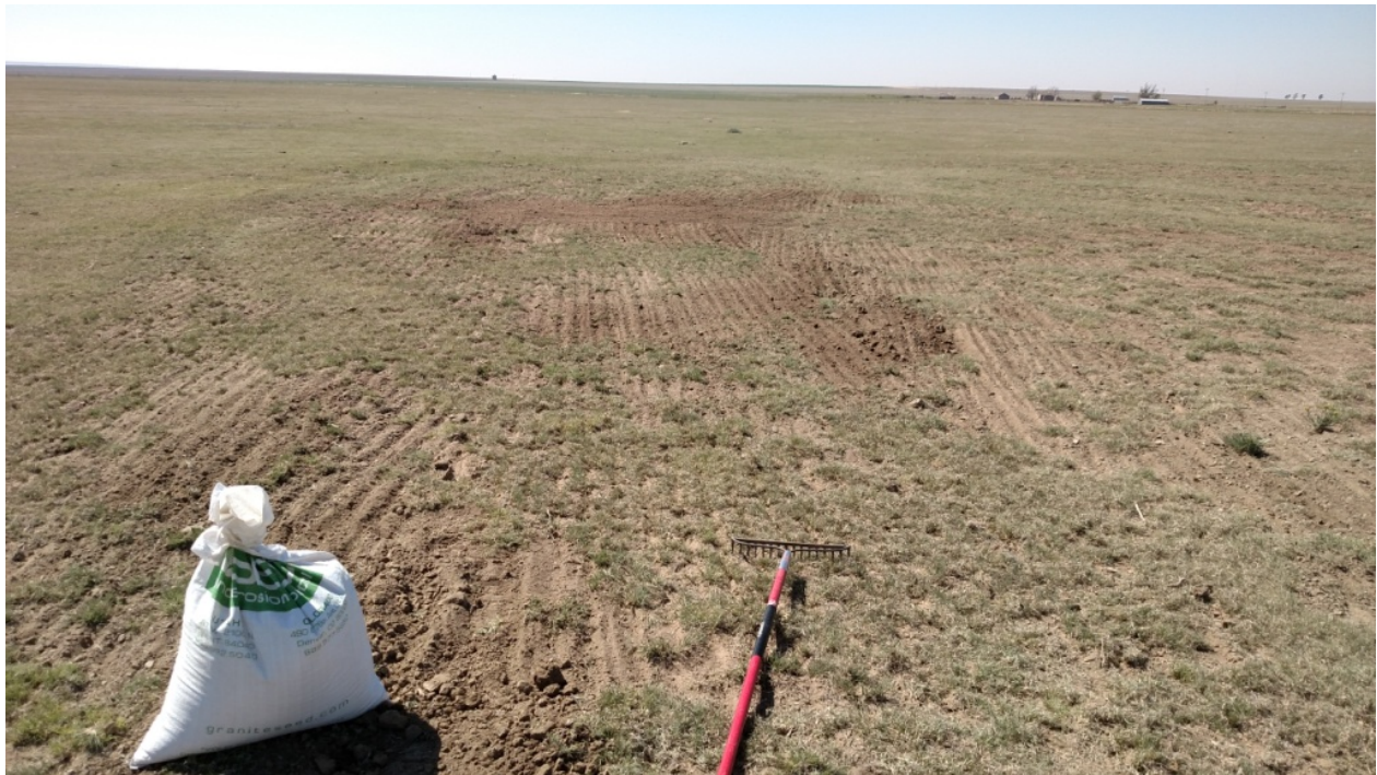
photo 9: Bare areas were decompacted, fertilized, and seeded.
