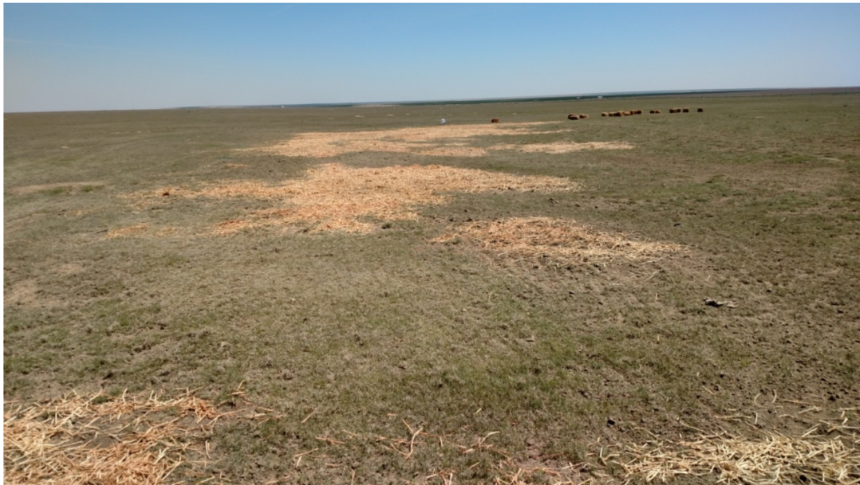
photo 11: Areas bare of vegetation covered with wood straw mulch approx 50% coverage.
