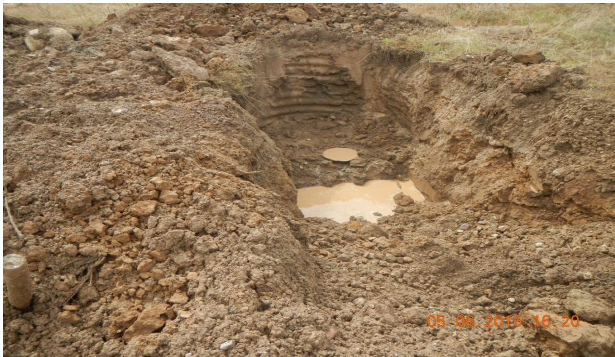
photo 19: Cellar ring has been removed. Conductor pipe found about 5ft. below the surface.
