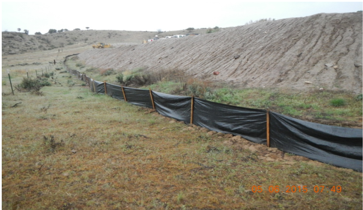
photo 5: Silt fence installed around the west side of the location.
