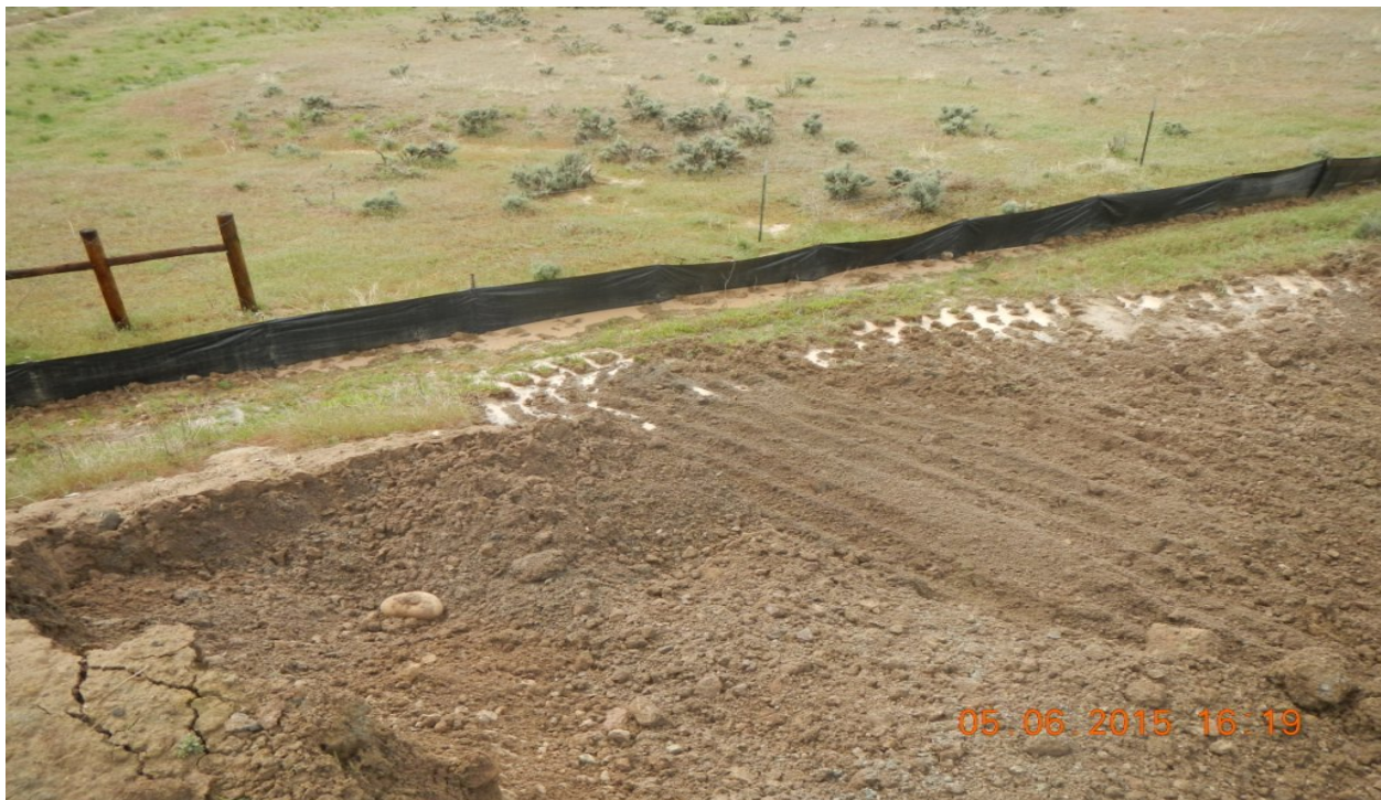
photo 18: West side of the location where silt fence is preventing sediment from running off site.
