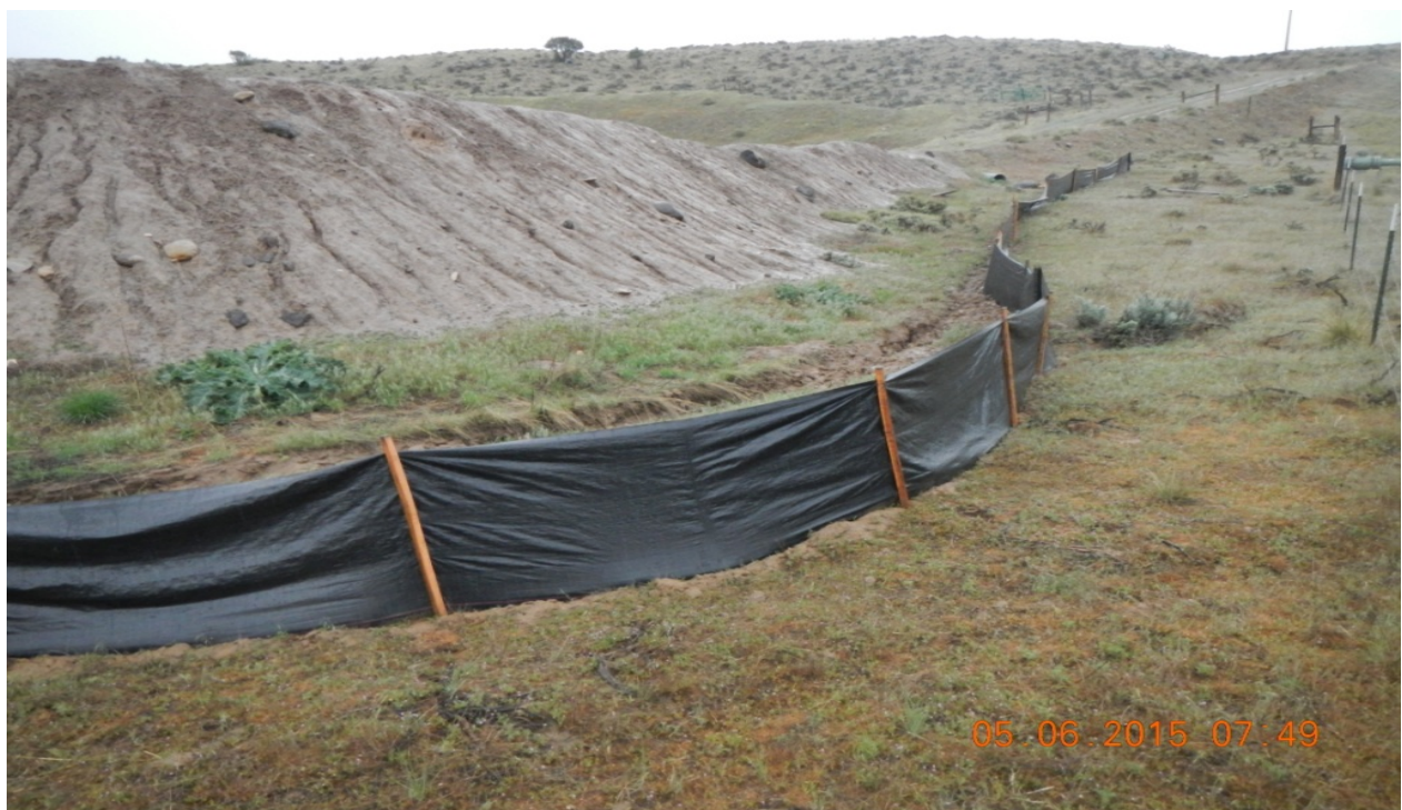
photo 6: Facing east, silt fence has been installed prior to excavation operations.
