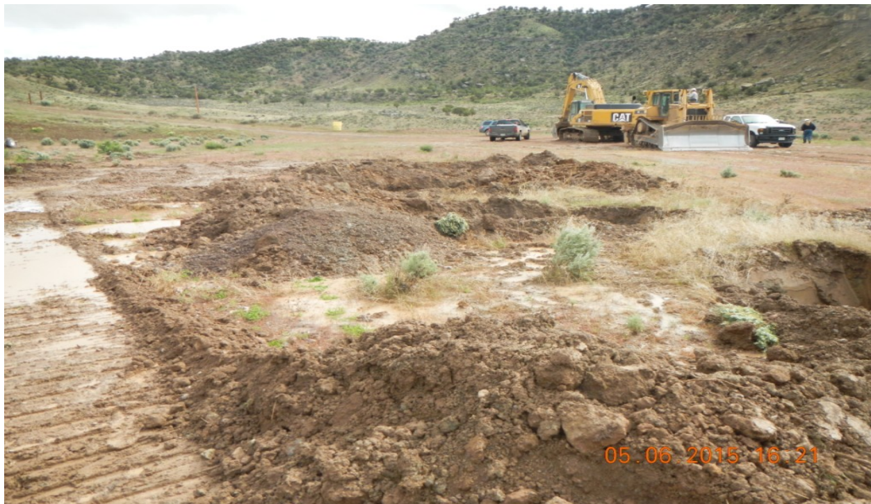
photo 20: Center of the location where 4 cellar rings have been removed.
