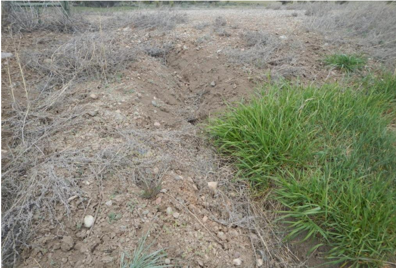
Photo 4. View of rill erosion from stormwater flows exiting the southern edge of the working area.
