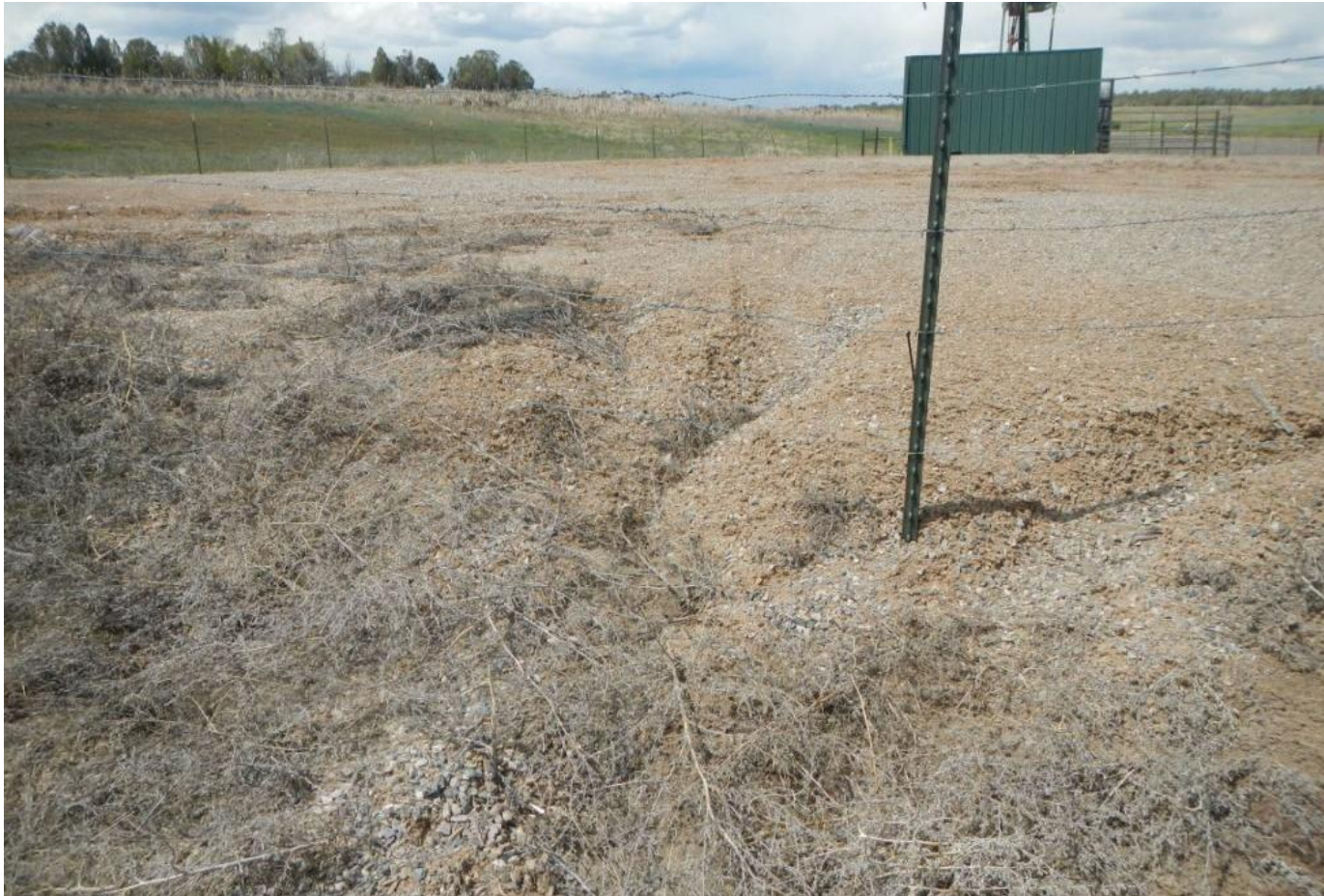
Photo 1. View of rill erosion from what appears to be stormwater flows exiting the southern edge of the working area of the well pad.
