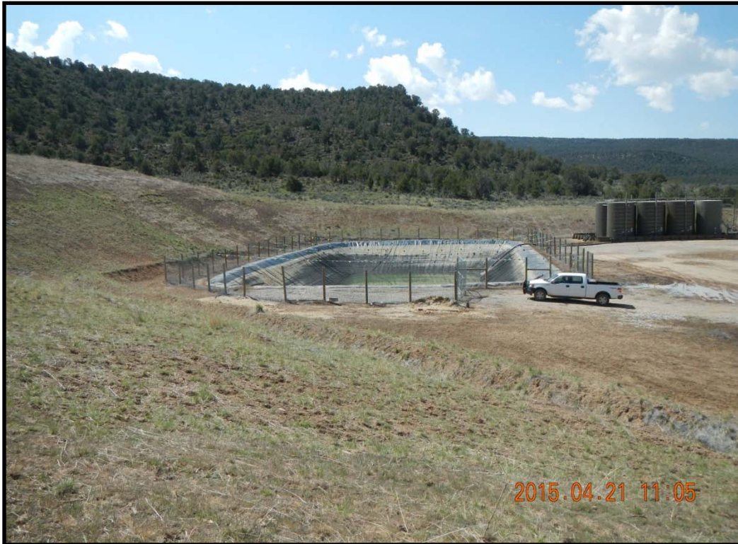
View of the multi-well pit. Looking west-southwest. Pit is fenced and colored flags are in place for bird protection.
