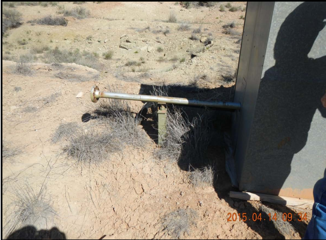
Disconnected piping from well to meter house.
