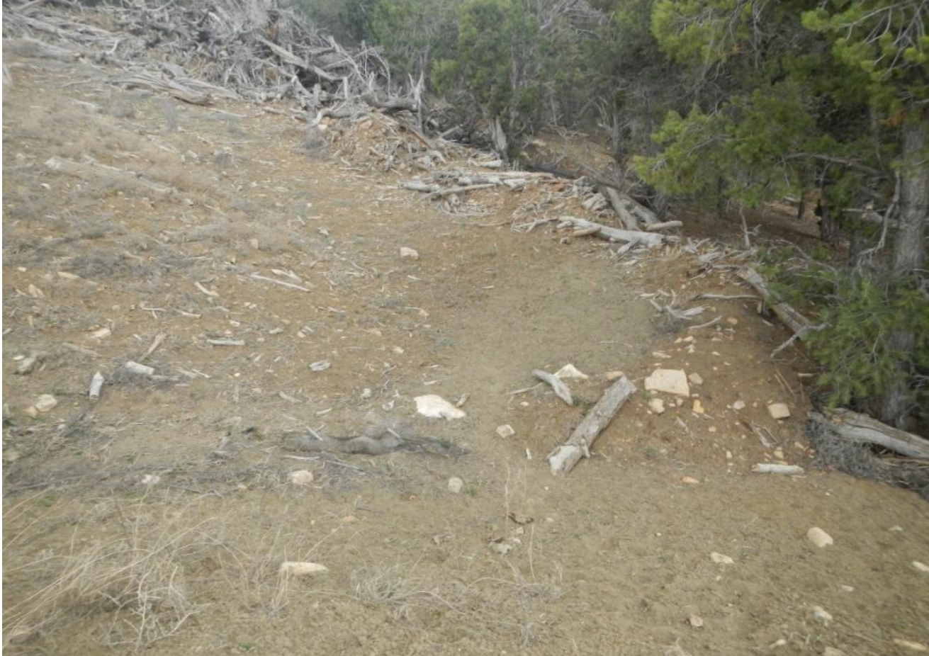
Photo 15. View of stormwater diversion in southeastern portion of project area that appears to be full of sediment.
