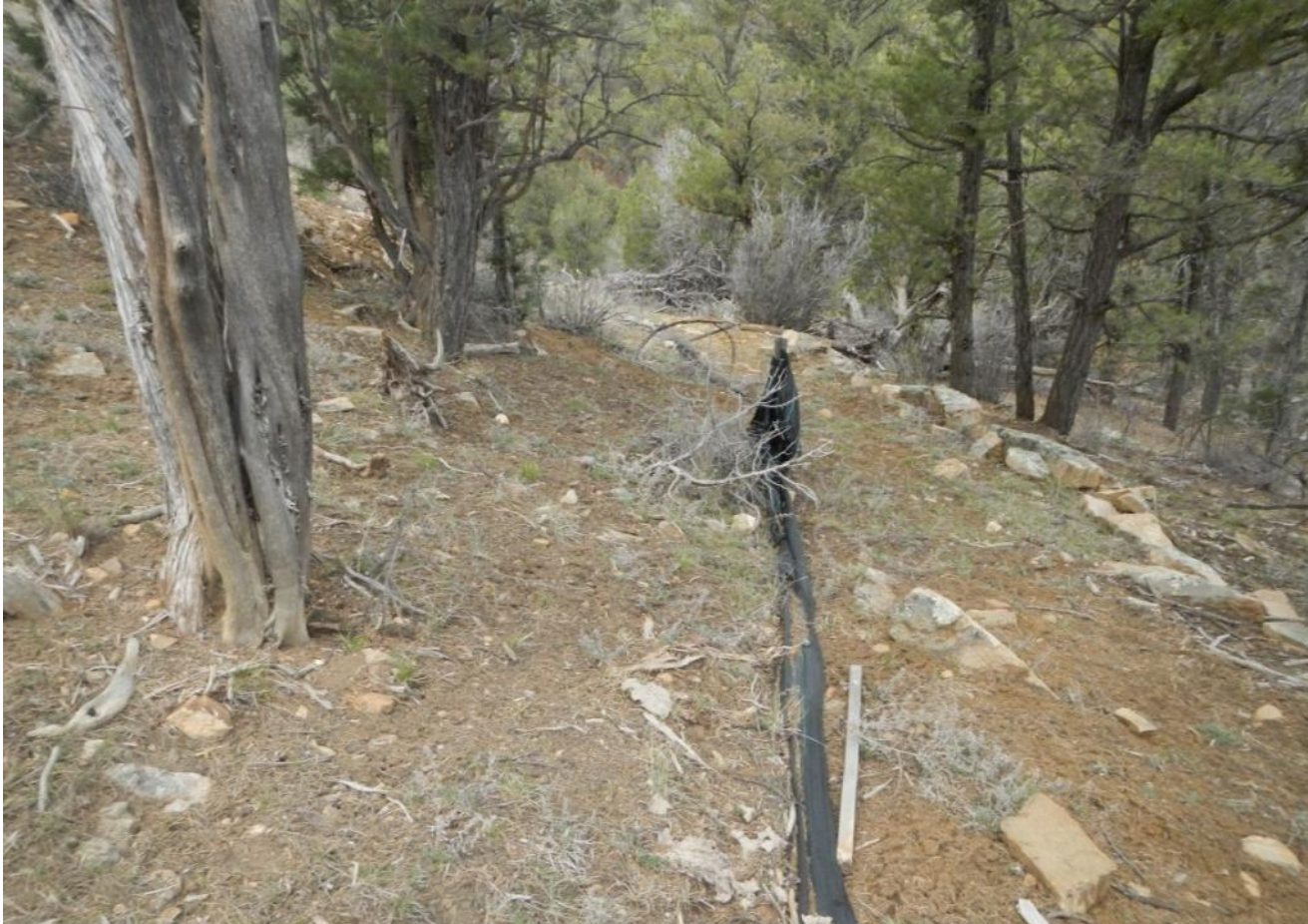
Photo 7. View of dilapidated silt fence that is installed around the perimeter of the project area.
