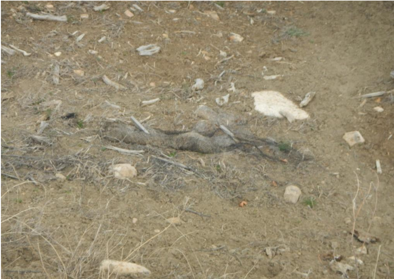
Photo 14. View of degraded straw wattle in southeastern portion of project area.
