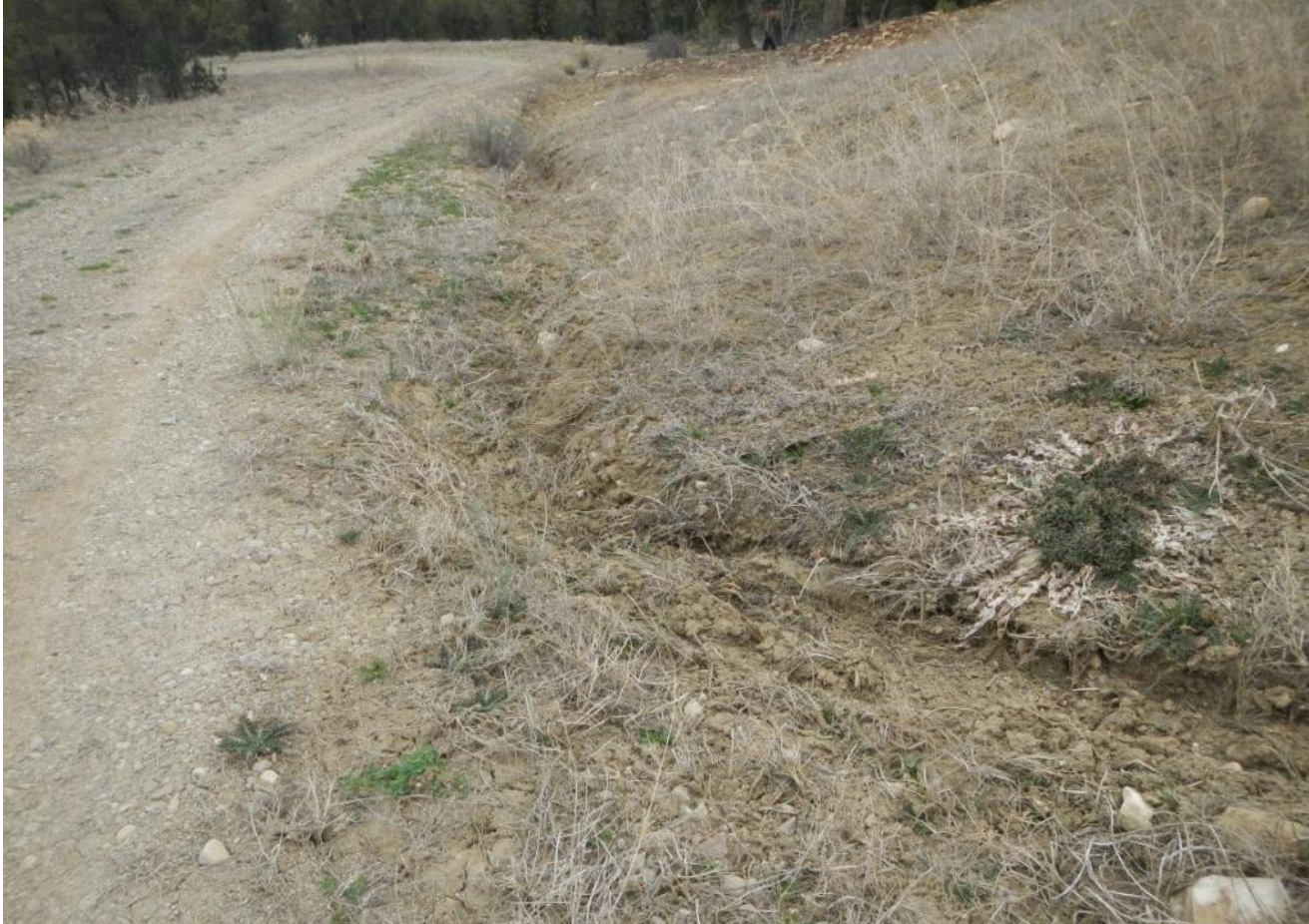
Photo 6. View of access road from well pad facing northward. Erosional channel is forming on the eastern edge of the access road from the well pad.
