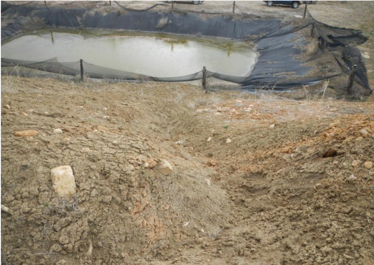
Photo 19. View of stormwater erosion toward pit from cut slope on eastern portion of well pad.
