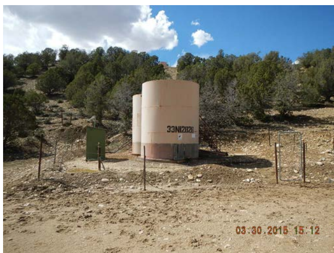
Battery (inadequate berm capacity)
