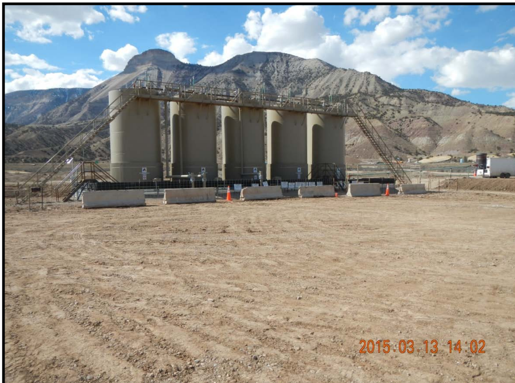
Tanks labeled and bermed. Clean pad. No staining observed, no weeds or junk.
