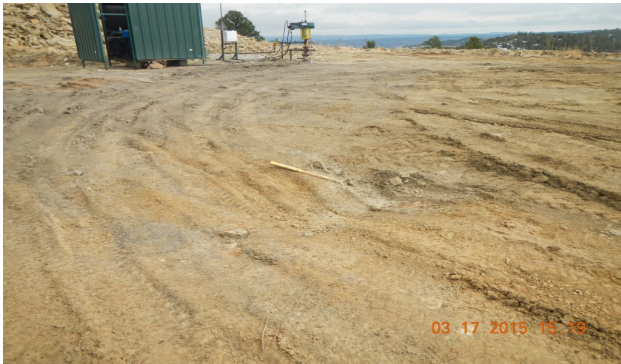
photo 3: Guy line anchor marker has fallen over.
