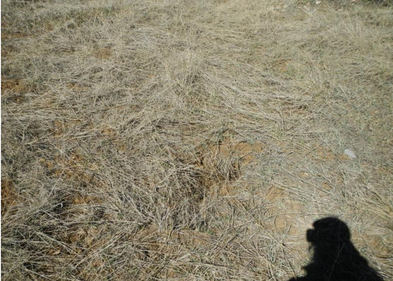
Photo 7. View of hole where it appears stormwater flows have eroded the well pad and begin to flow beneath the ground.
