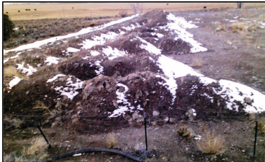
Viewing west: E&P Landfarm strip and adjacent berm & ditch stormwater BMPs.
