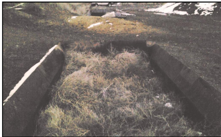
Viewing East : open receptacles containing miscellaneous debris: weeds, dirt, oily debris & stormwater.
