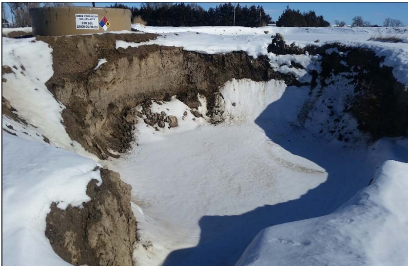
Photo 1 – Photo of open excavation for remediation of oil skim pit
