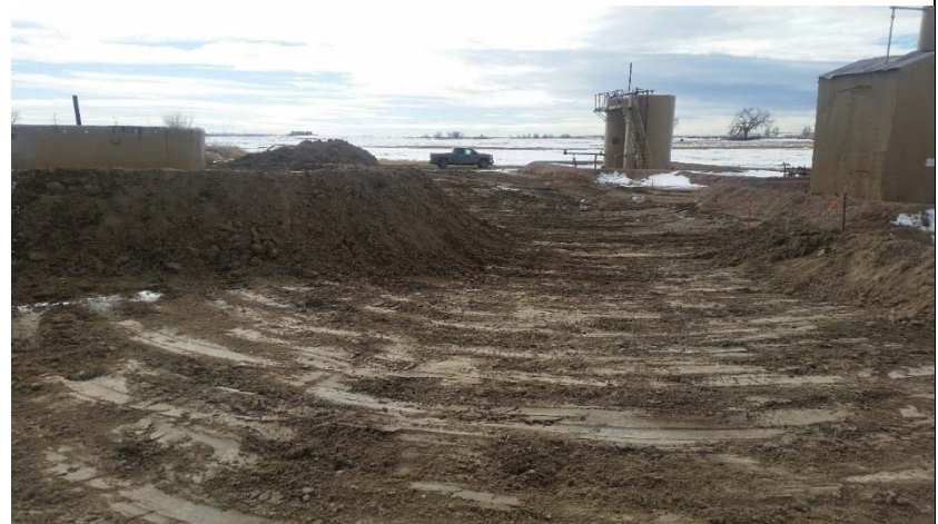
Photo 2 – Photo of recontoured area from pit excavation and backfill (looking NNE)
