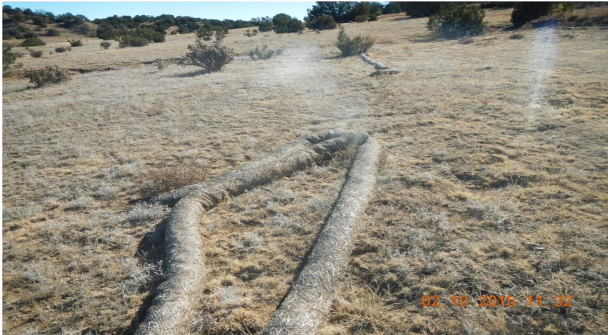
photo 9: Waddles are displaced at the north side of the location.
