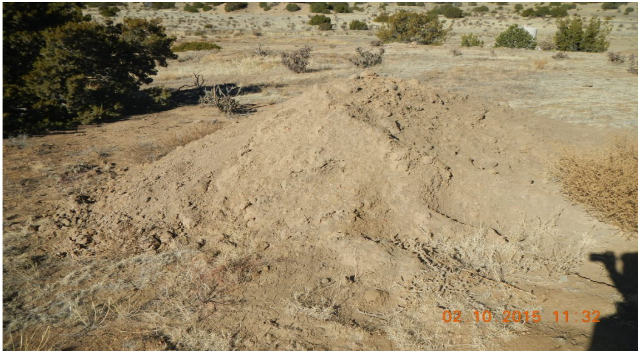
photo 8: Soil stockpile at the southwest corner of the location is not stabilized.
