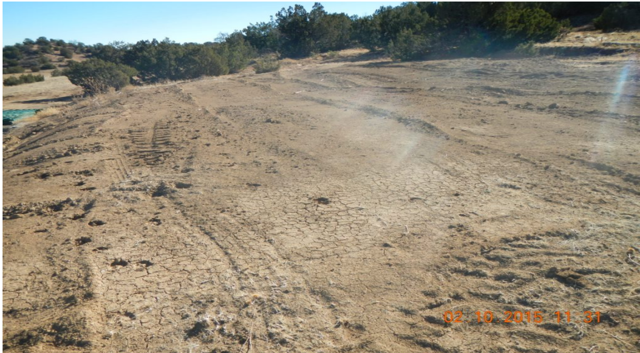
photo 7: The area on the south side of the location has not been reclaimed and is susceptible to erosion.
