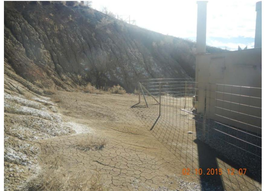
Erosion rills of cut slope wall being used for back wall of tank berm.
