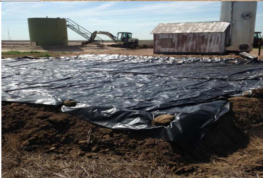
**Subject:** A plastic lined containment cell was constructed for the impacted soils excavated from the former skim pit.
