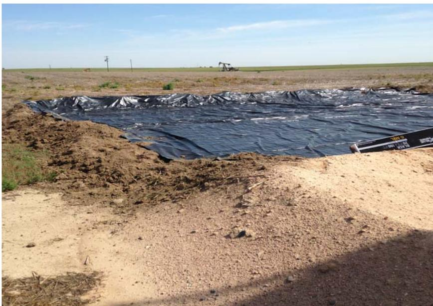
**Subject:** The plastic lined containment for the impacted soils was located on the north side of the vertical treater berm at the S.J. Warren tank battery location.
