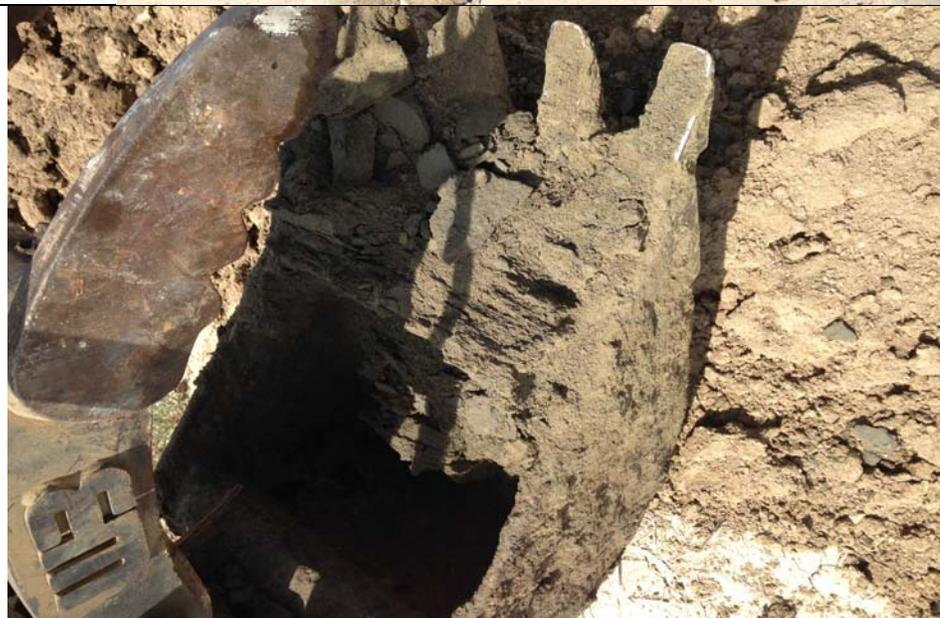
**Subject:** Stratified, sandy shale was encountered in the bottom east side of the excavation at approximately 19 feet below ground surface. Odor and staining diminished at this depth.
