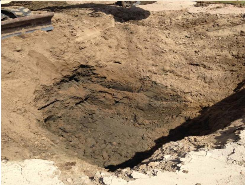
**Subject:** Olive gray staining was noted in some of the soils in the excavation. Impacted materials were excavated from the former S.J. Warren skim pit and were placed in the lined secondary containment cell pending treatment.
