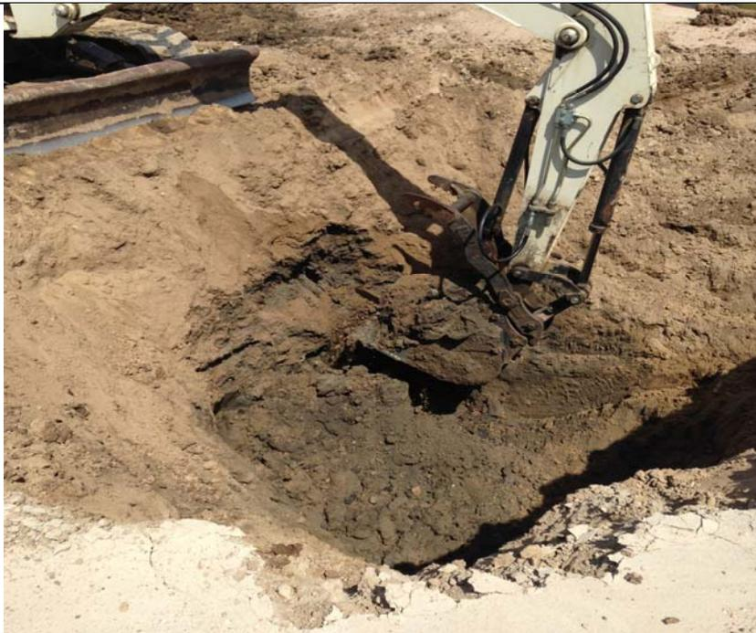
**Subject:** The excavation of the former skim pit was advanced to a maximum depth of 19 feet on the east side closest to the active produced water pit. Olive gray staining was observed in the soils in the sidewalls and base of the excavation.
