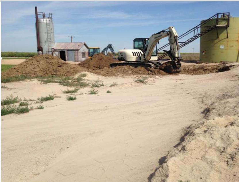
**Subject:** An Ingersoll Rand trackhoe excavator was used to excavate the impacted soil from the former skim pit at the S.J. Warren site.
