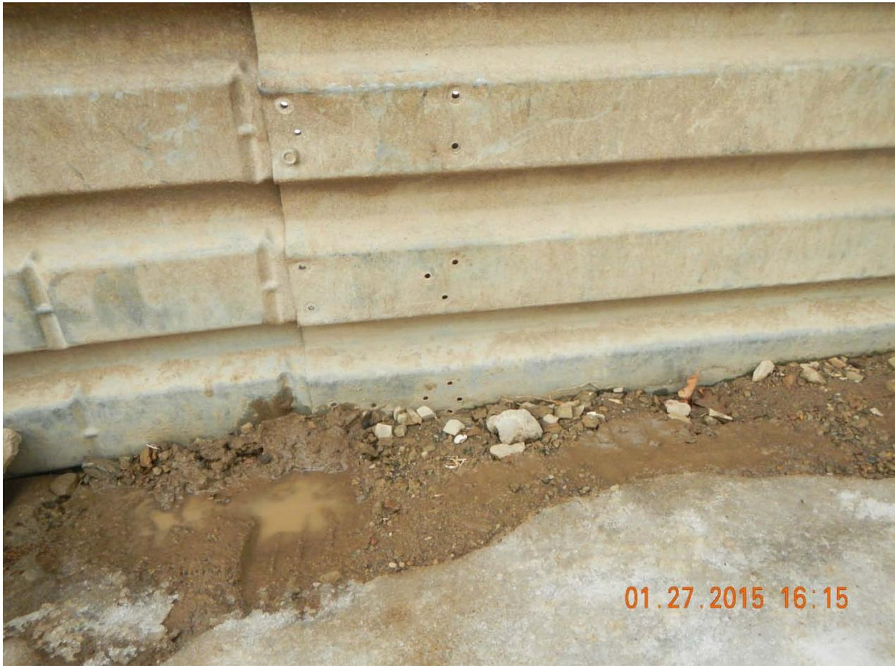
Bolt together berm with no liner and
