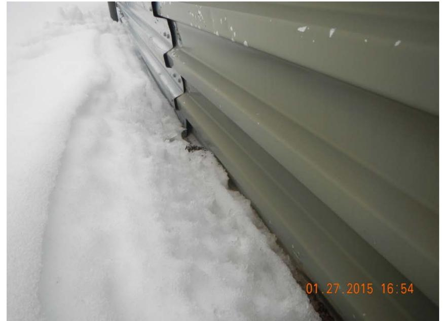
Day lighting in corner of berm where connected to adjacent berm for 400 bbl tank.
