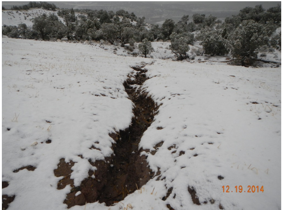
Erosion from drain outlet on reclaimed area.
