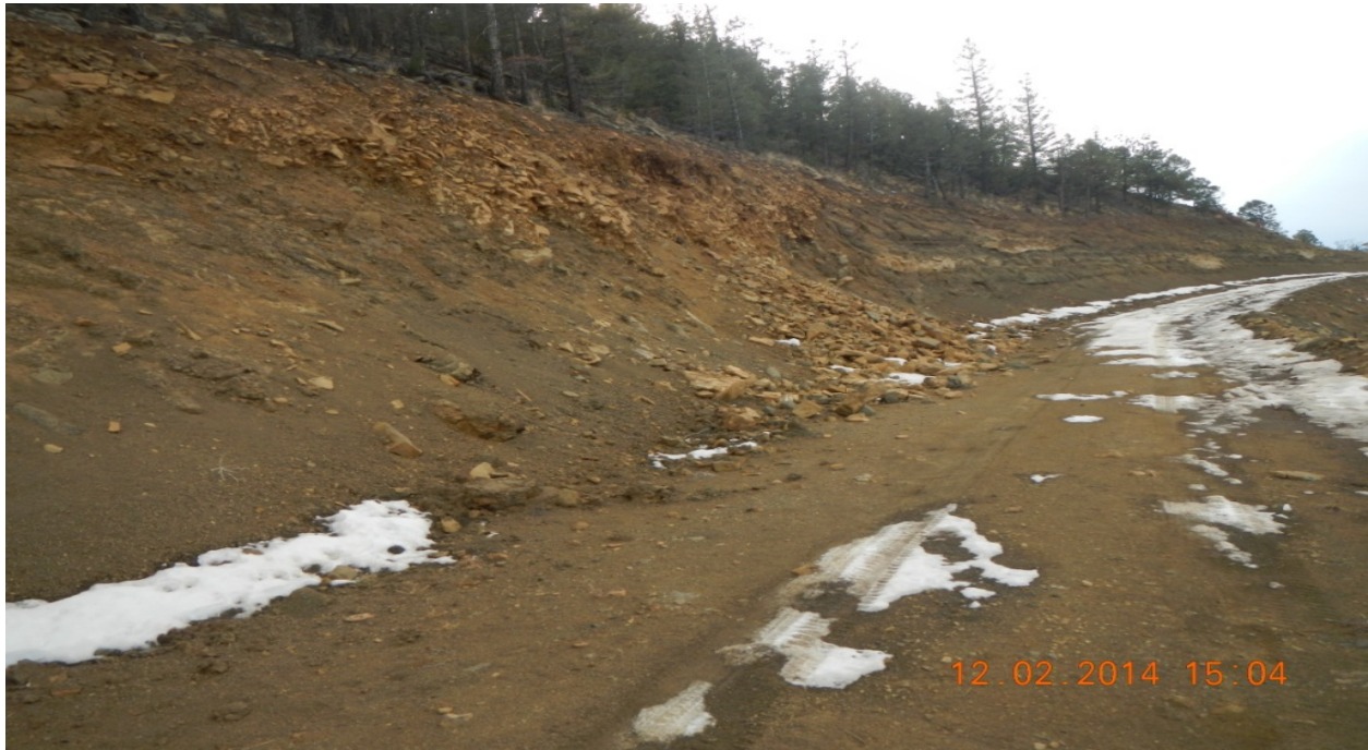
photo 15: Steep cut is not stable. Rocks are falling down onto the road.
