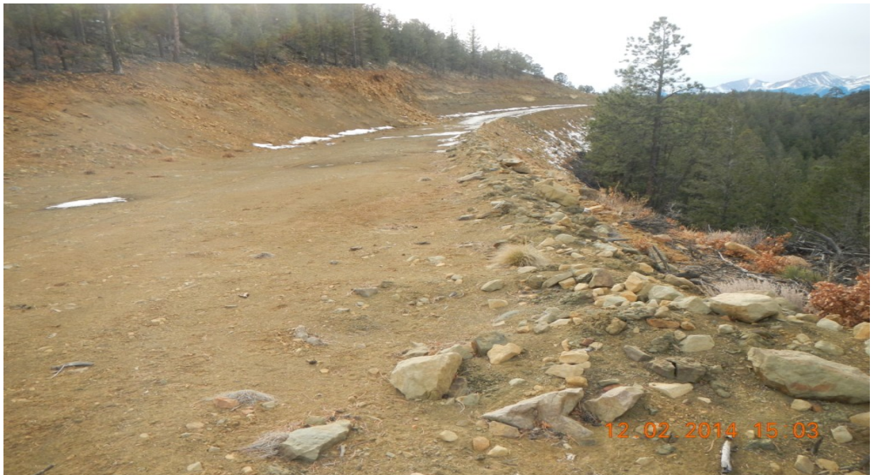
photo 14: Facing West along the access road. Severe cut into the mountain face.
