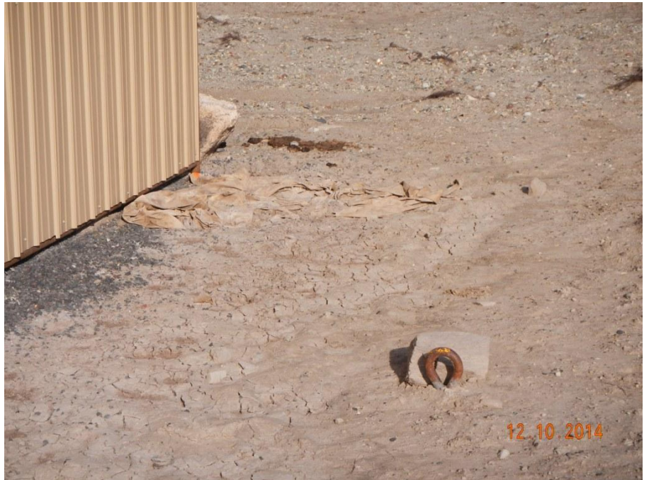
Unmarked deadman, trash and sediment run-on.
