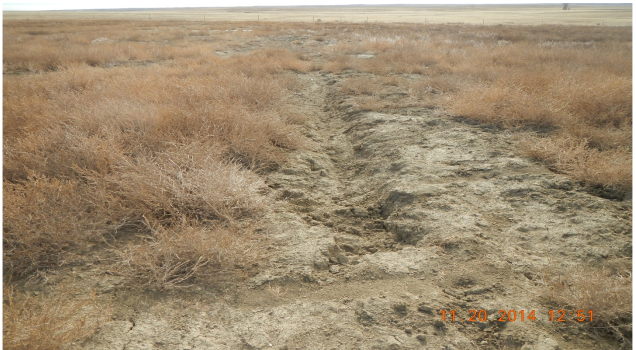
photo 8: Erosion occurring through the center of the location has created a ditch.
