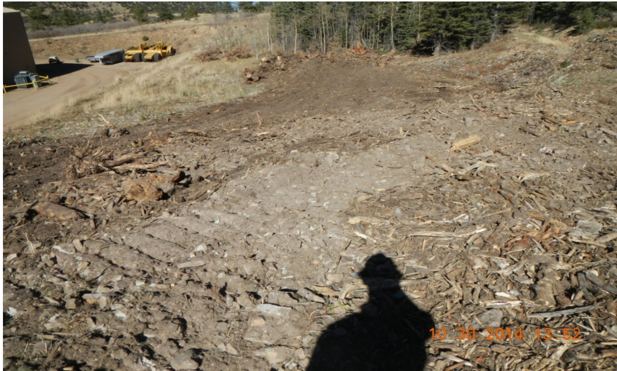
Ground disturbance on East side of location creates erosion potential
